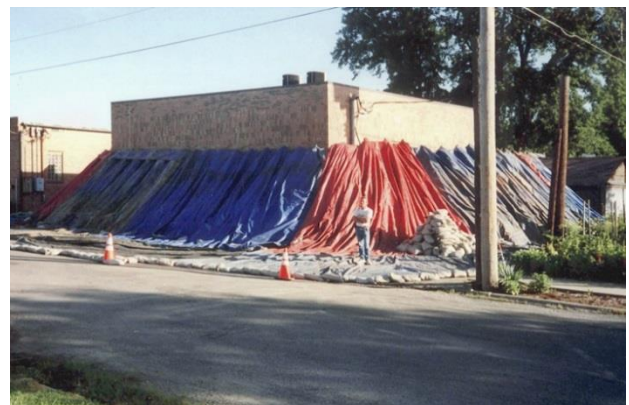
Protecting critical telecommunications infrastructure
