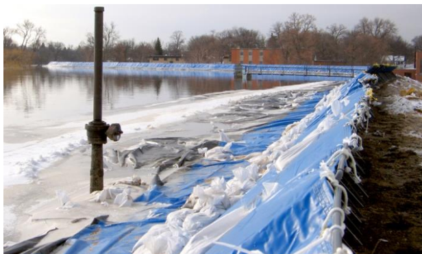
Levee extension in Fargo, North Dakota
