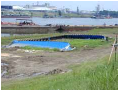
Figure 3-177. Portadam structure prior to removal
