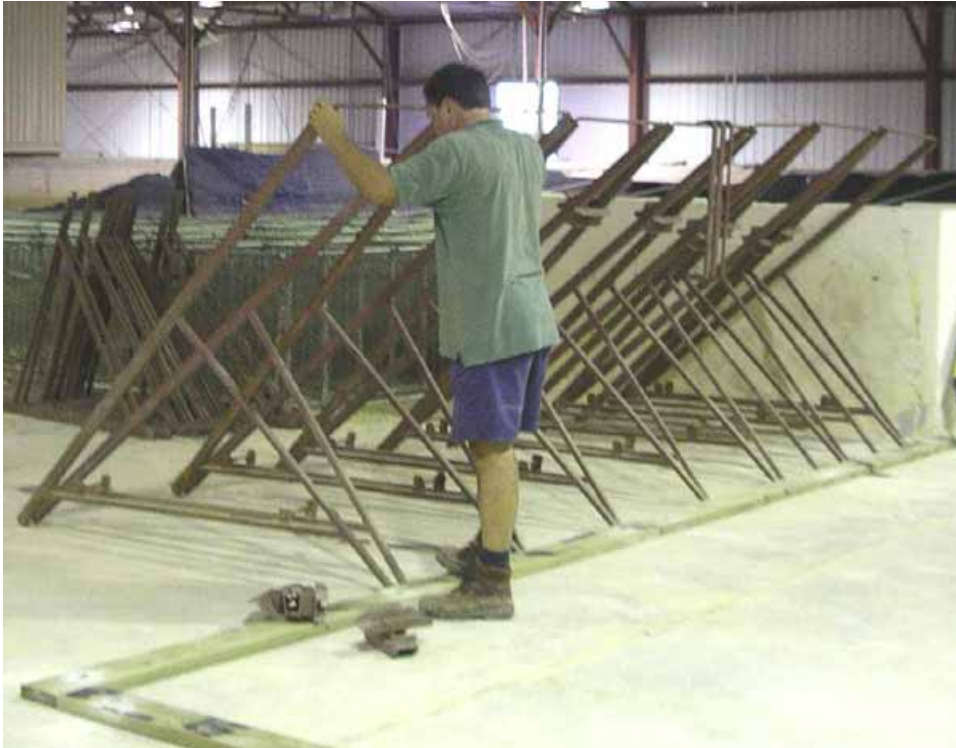
Figure 2-191. Beginning frame installation from right abutment wall
