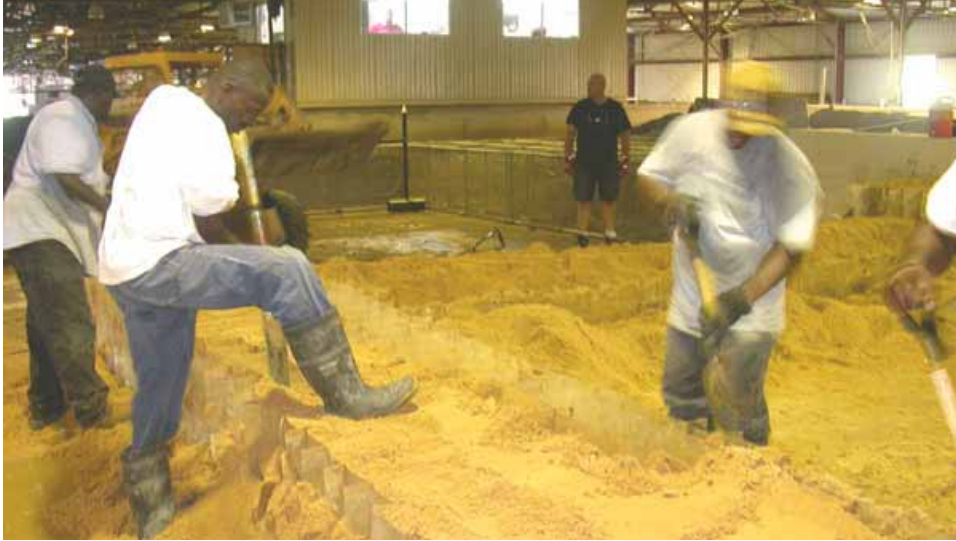
Figure 2-178. Continuation of sand removal using shovels
