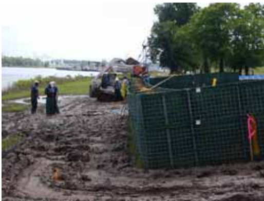
Figure 3-76. Filling top row units with sand
