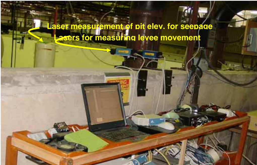
Figure 2-5. Seepage and displacement data retrieved by data acquisition system
