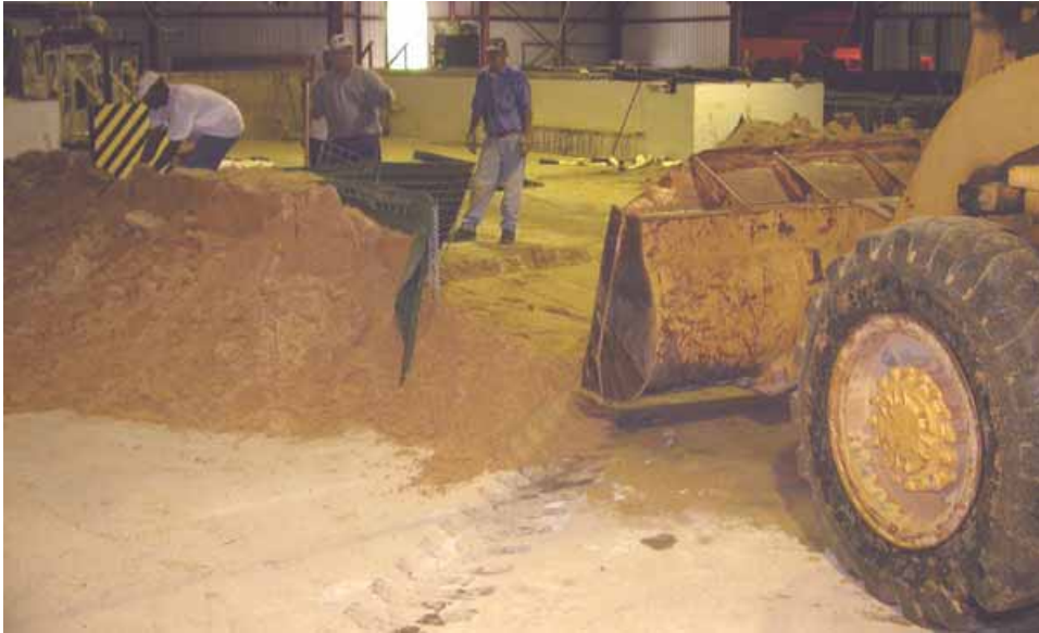
Figure 2-95. Removing sand pile
