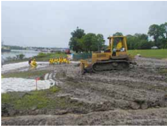
Figure 3-40. Area being backdragged to reduce mud
