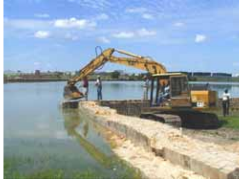
Figure 3-125. Trackhoe replacing sand field
