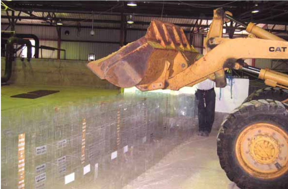
Figure 2-113. Begin sand fill on left wall
