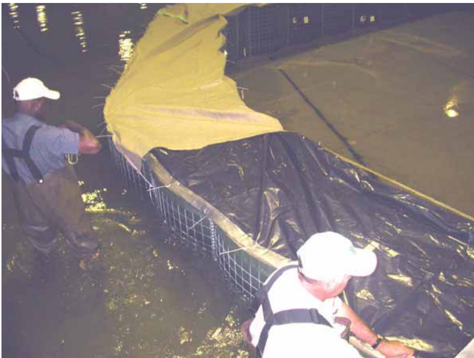
Figure 2-75. Securing with cable ties
