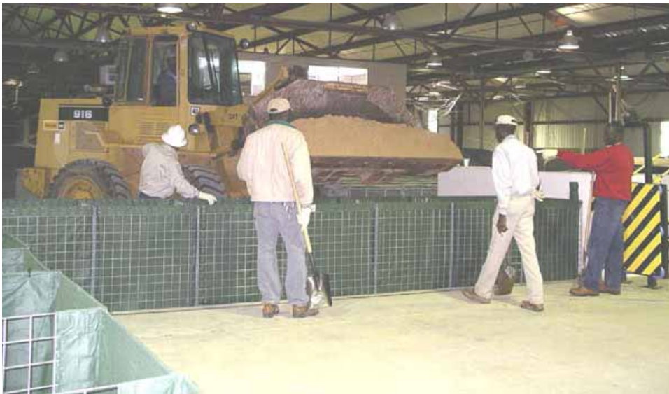
Figure 2-53. Filling with sand
