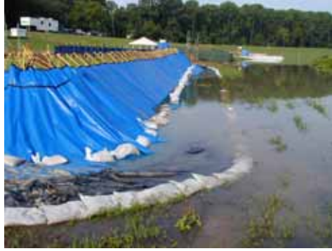
Figure 3-159. 5 June 2004, 0.3 ft of water against structure
