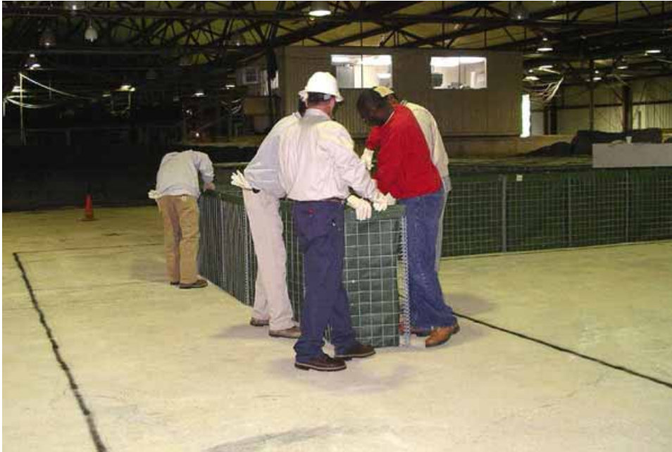
Figure 2-47. Expanding and positioning units
