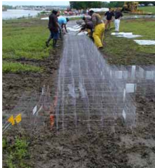
Figure 3-112. Filling of west tieback section units
