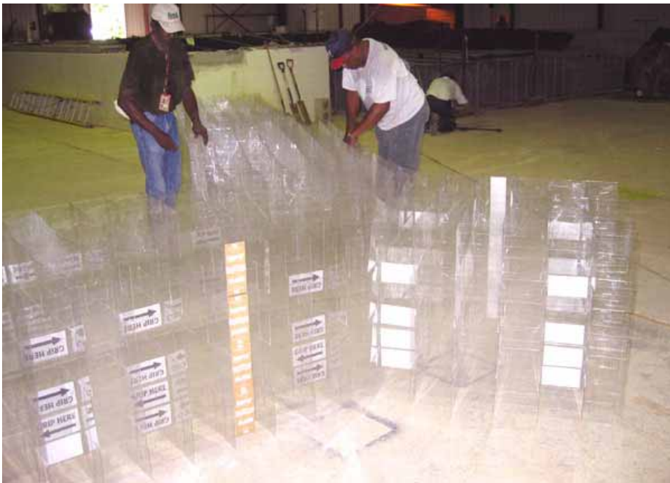
Figure 2-110. Top (fourth) grid layer installed along center wall/left wall buttress as viewed from pool side
