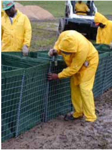
Figure 3-72. Installation of joint pins
