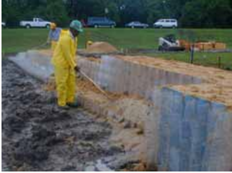
Figure 3-109. Installation of tieback section
