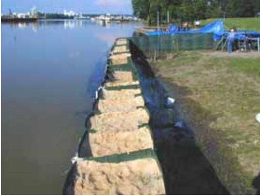
Figure 3-86. 10 June 2004, 3.5 ft of water against structure
