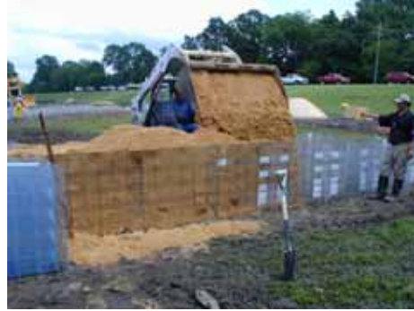
Figure 3-110. Installation of riverward face and tieback section
