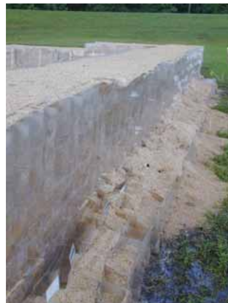
Figure 3-116. Riverward face of completed structure
