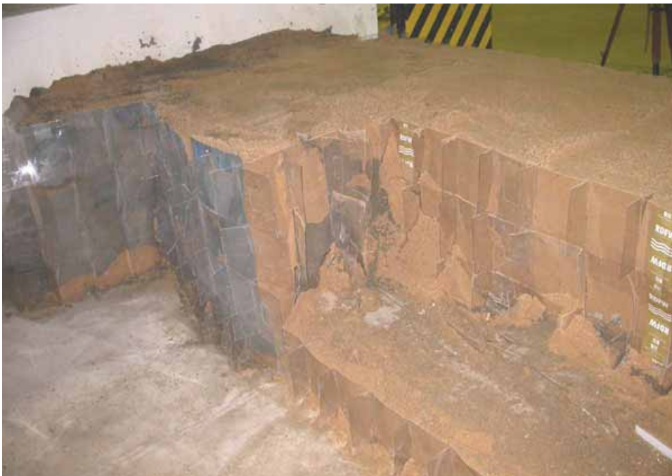
Figure 2-123. Right concrete wall abutment completed sand and mixture fill, viewed from pool side
