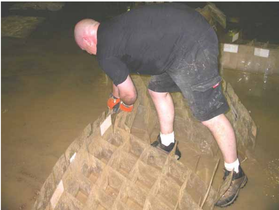
Figure 2-176. Disassembling grid unit for future reuse
