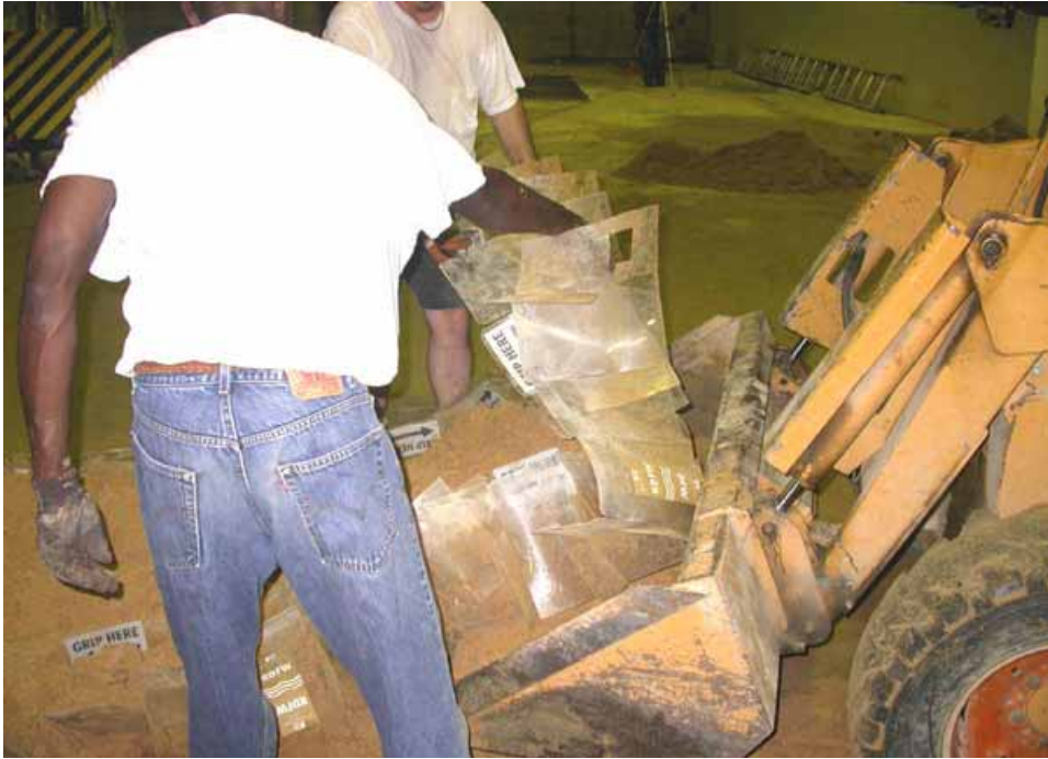
Figure 2-182. Removing grid unit/sand combination
