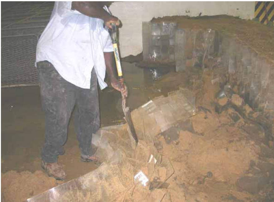
Figure 2-164. Shoveling out sand/cement mixture from toe grid units and pulling out grid
