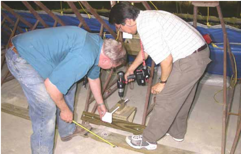
Figure 2-213. Installing one of laser targets
