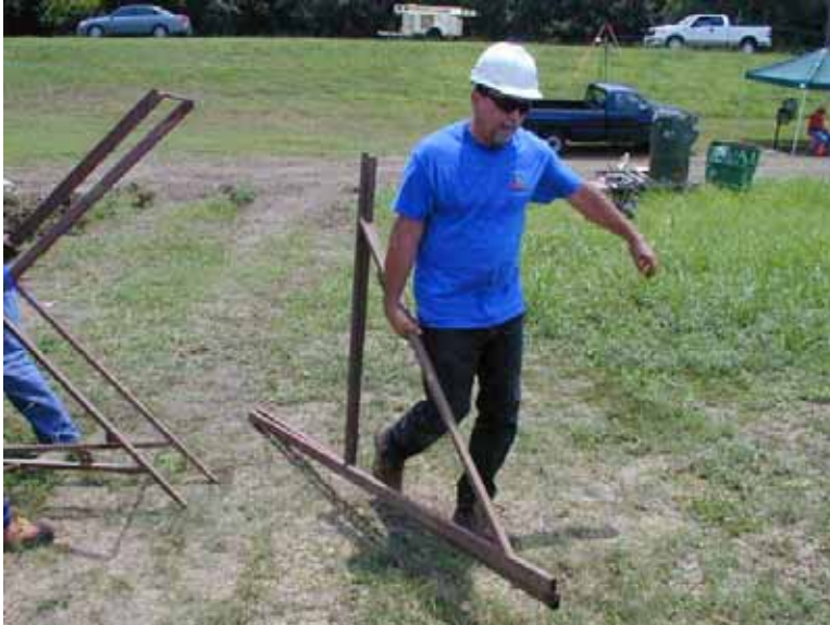
Figure 3-181. Carrying frame members to staging area
