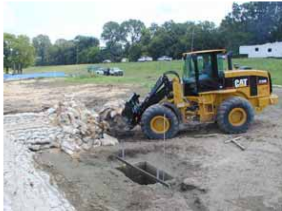
Figure 3-62. Sandbags removed by front-end loader
