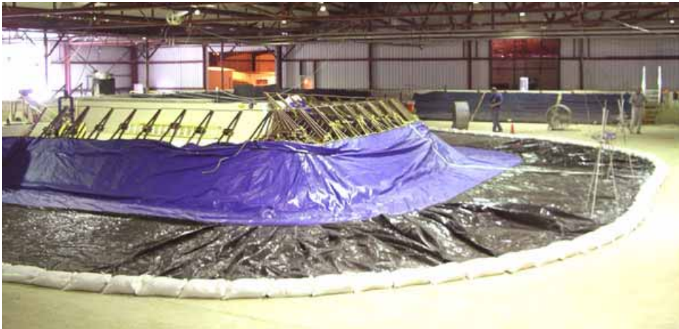
Figure 2-211. Portadam® levee construction completed
