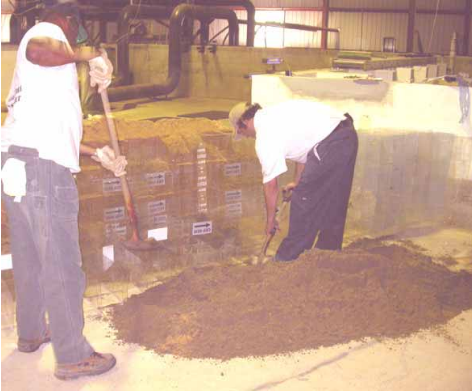
Figure 2-116. Shoveling mixture into left wall toe grid cells
