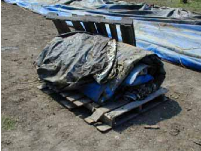
Figure 3-188. Liner placed on pallet
