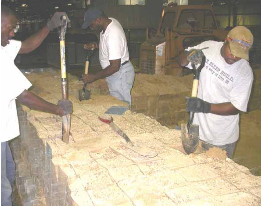
Figure 2-169. Removing sand using shovels
