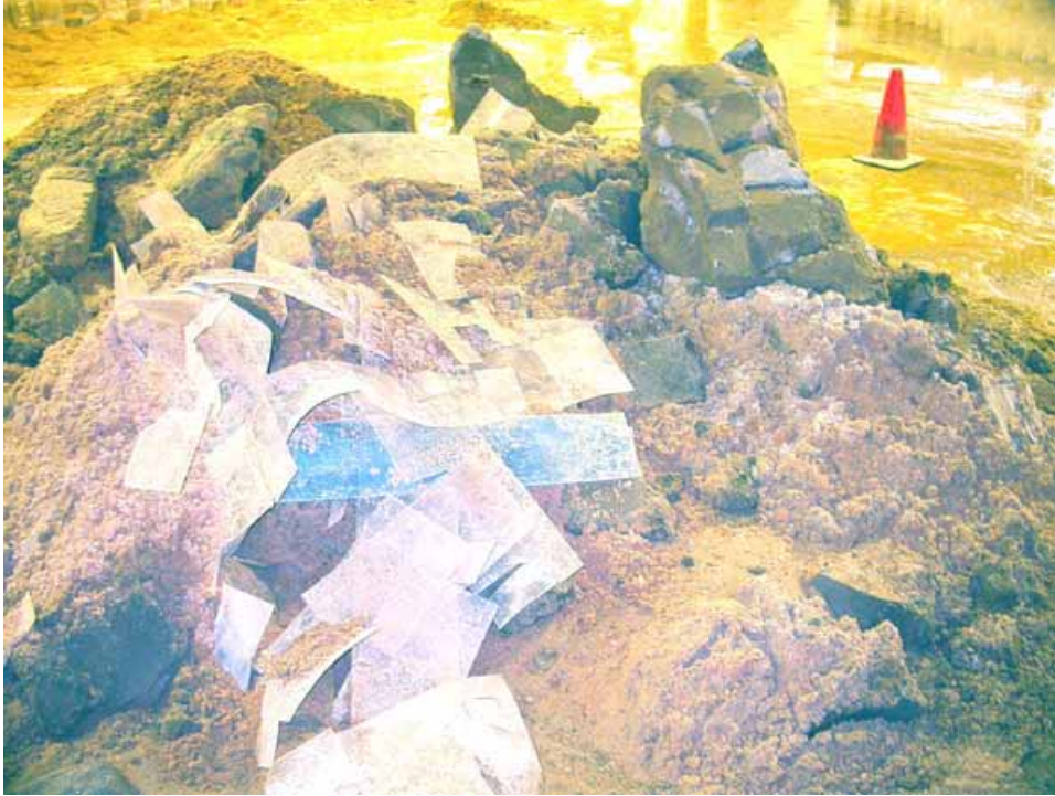
Figure 2-184. Nonreusable grid units, sand, and sand/cement mixture ready for disposal
