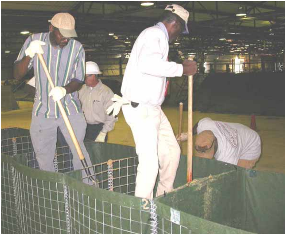
Figure 2-55. Leveling and compacting sand within each unit
