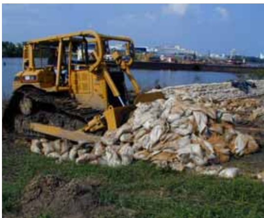
Figure 3-63. Bulldozer piling up sandbags
