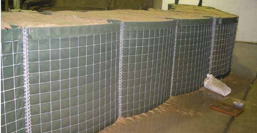
Figure 2-88. Added sandbag along left wall
