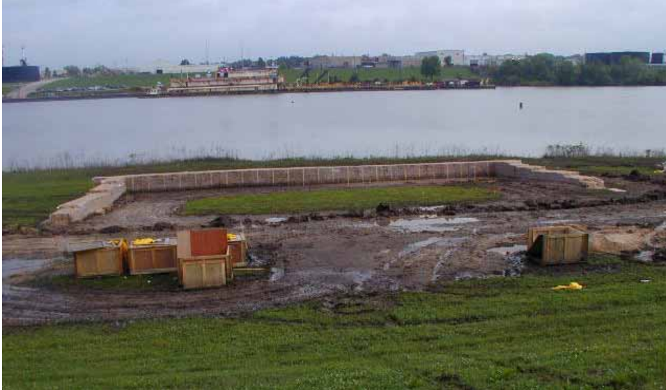
Figure 3-117. Completed RDFW structure
