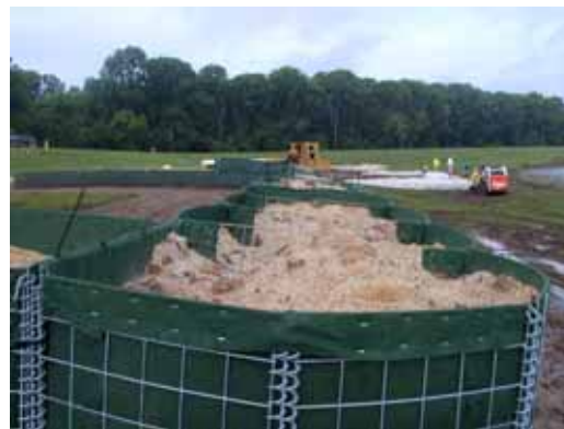
Figure 3-77. Sand fill in top row units
