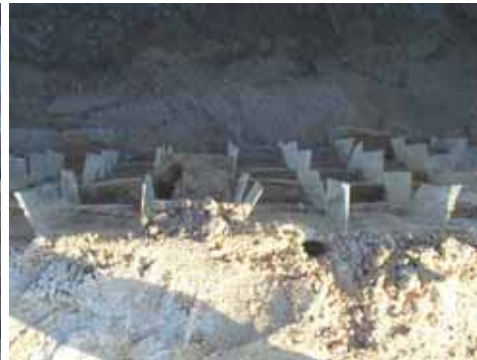
Figure 3-123. Shifting of units (view down front edge from top)
