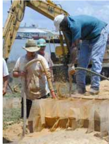
Figure 3-134. Sand removal from RDFW structure with water hose and compressed air
