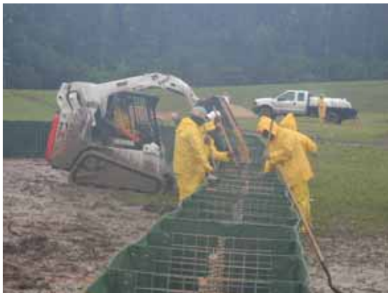
Figure 3-74. Filling base row with sand
