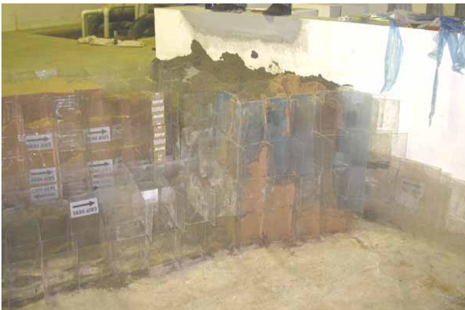
Figure 2-117. View of left concrete wall abutment from pool side
