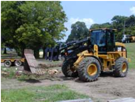
Figure 3-189. Loading Portadam frame members and hardware onto trailer
