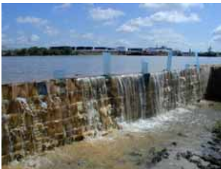
Figure 3-130. Final overtopping of RDFW structure
