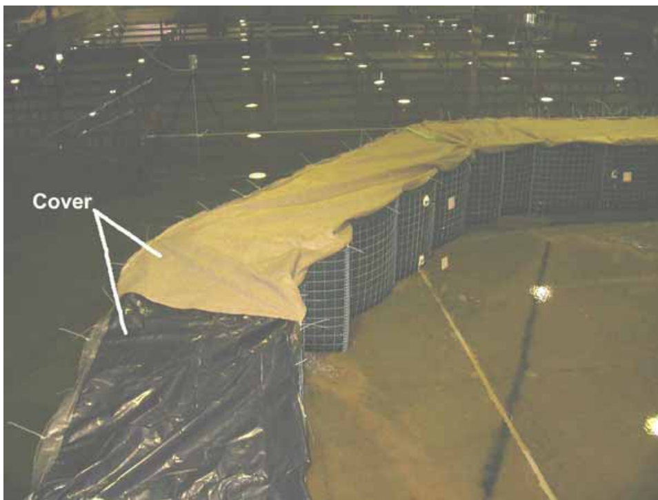
Figure 2-79. View of left and center walls
