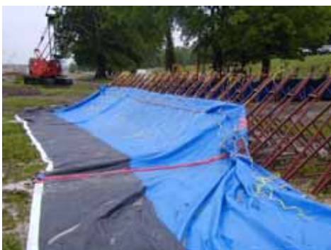
Figure 3-151. Liner membrane tied to support frame
