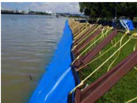
Figure 3-162. 8 June 2004, 2.7 ft of water against structure
