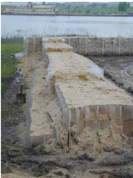
Figure 3-115. Sand fill in completed structure
