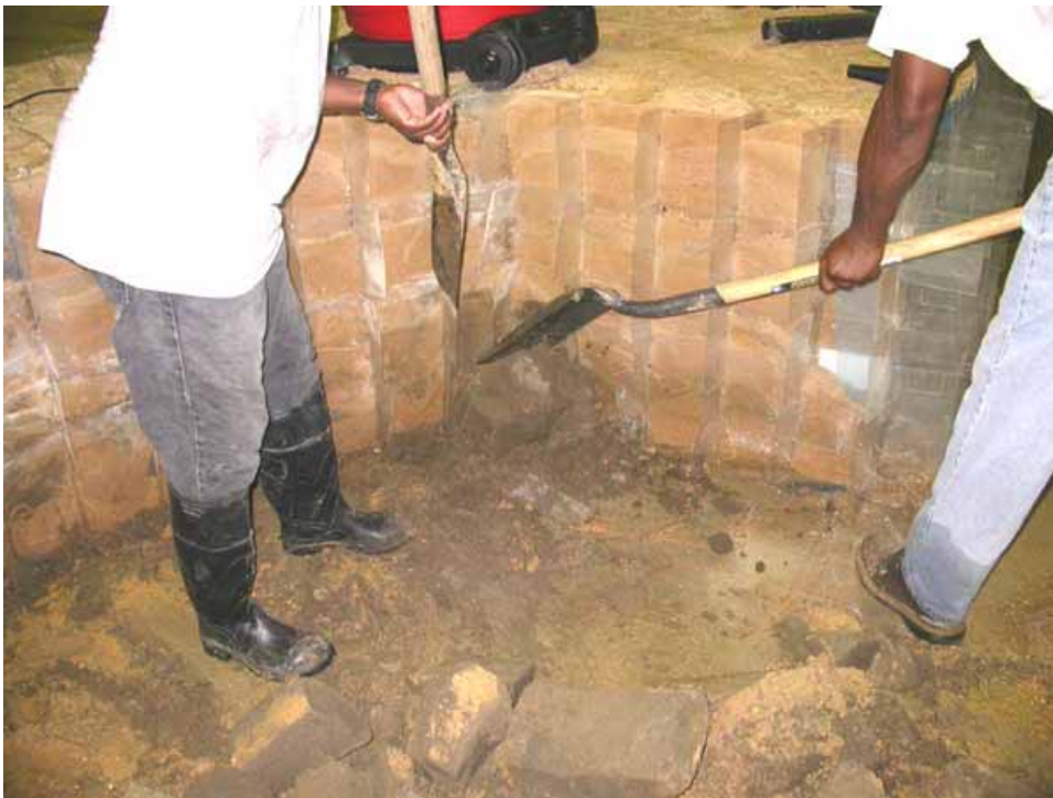
Figure 2-166. Cleaning out remaining toe grid materials
