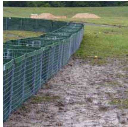
Figure 3-71. Structure constructed on graded ground and grass/weeds
