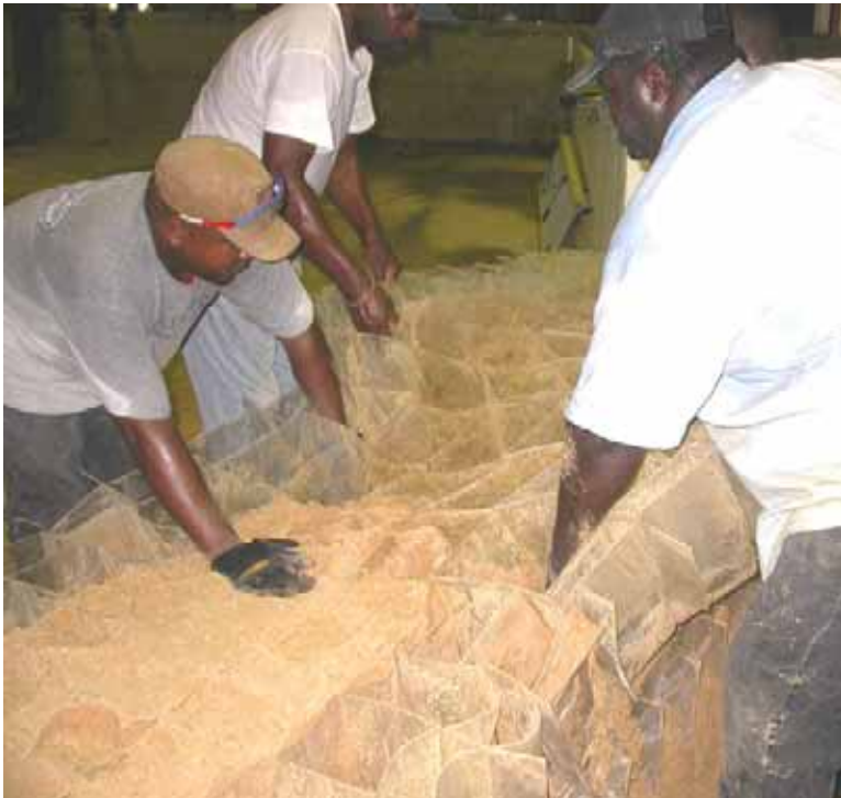
Figure 2-172. Pulling grid unit in an upward fashion
