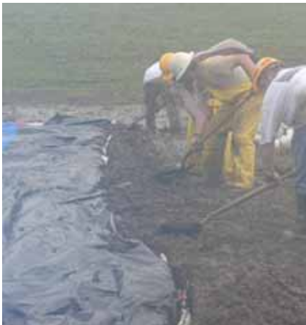
Figure 3-154. Burying liner leading edge
