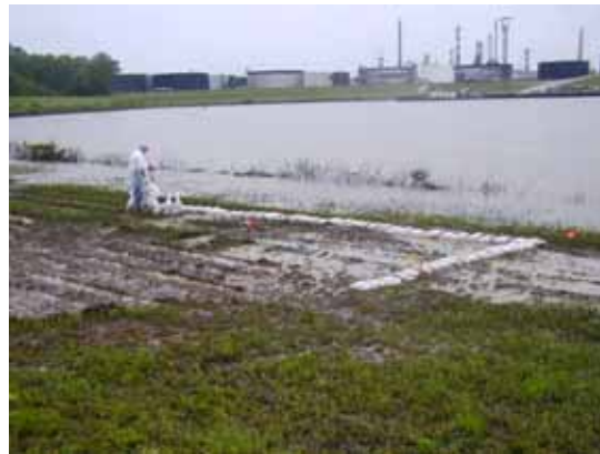
Figure 3-35. Laying first row of bags
