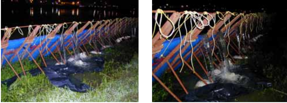
Figure 3-174. Overtopping of Portadam structure
