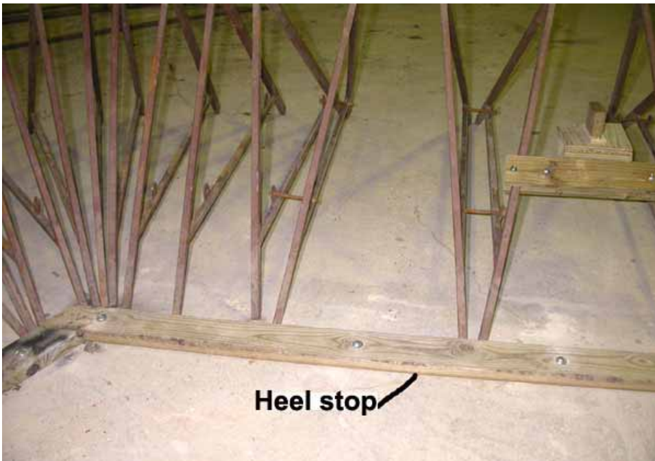
Figure 2-190. Frame 2 x 6 heel stop
