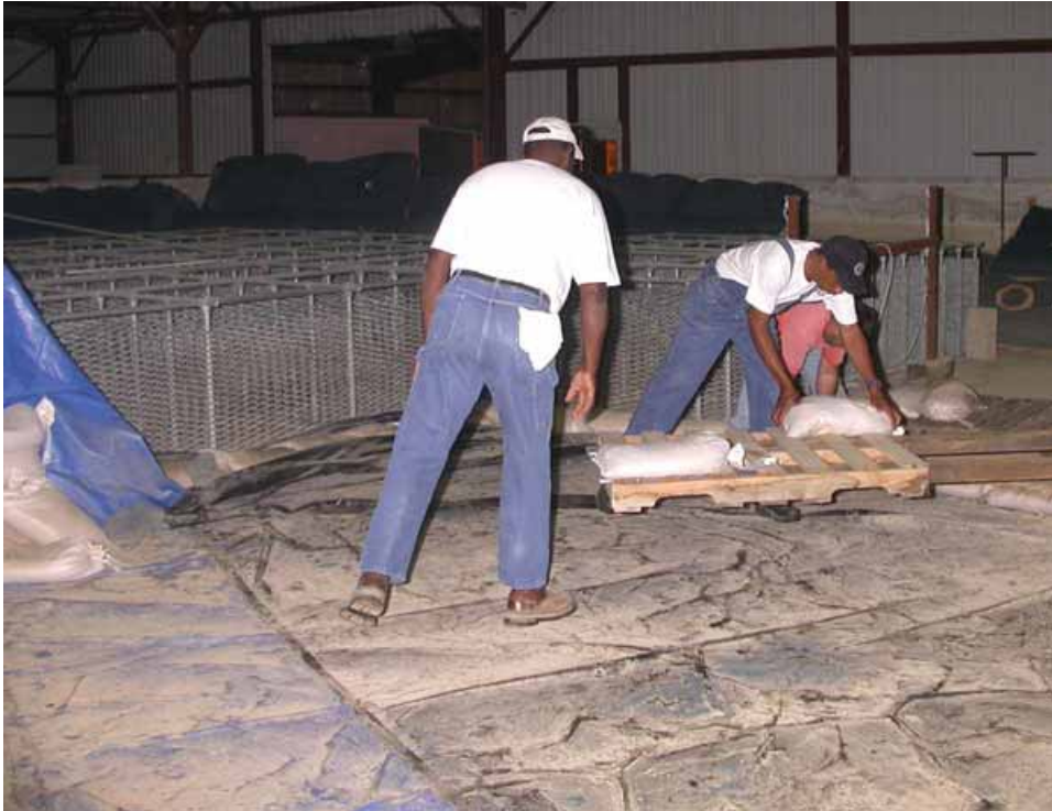
Figure 2-244. Removing and restacking periphery sandbags
