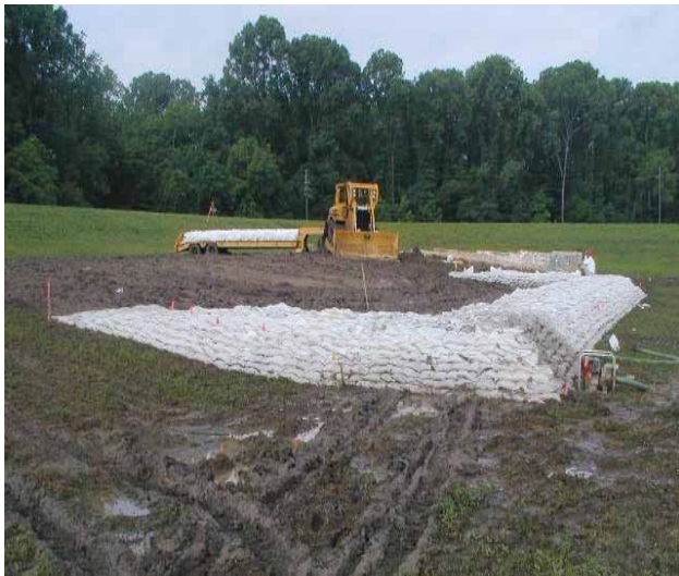
Figure 3-42. Completed 3-ft structure
