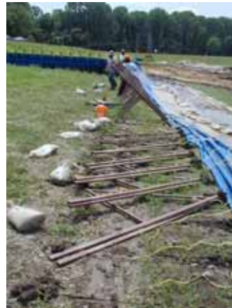
Figure 3-179. Disassembling supporting frame (bolts and clamps)
