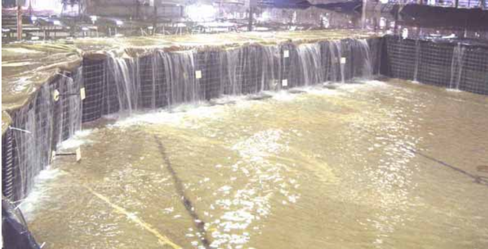
Figure 2-84. Overtopped levee structure, view from left wall
