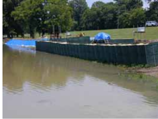
Figure 3-81. 5 June 2004, 0.3 ft of water against structure
