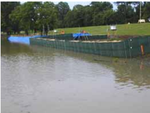
Figure 3-82. 6 June 2004, 1.3 ft of water against structure
