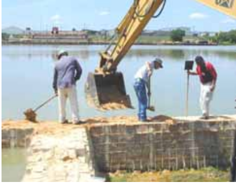
Figure 3-124. Replacing sand washed out or lost from shifted units
