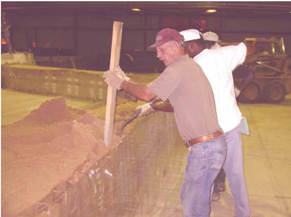
Figure 2-114. Tamping sand into cells along center wall, viewed from pool side
