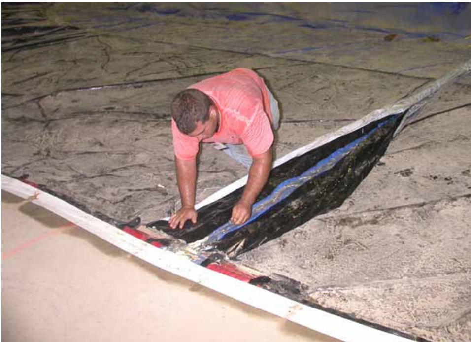
Figure 2-245. Unhooking and separating two vinyl tarp sections
