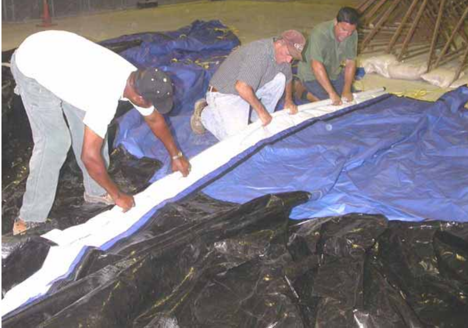
Figure 2-202. Rolling seam
