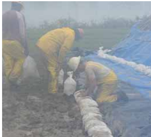
Figure 3-155. Placing sandbags on liner leading edge
