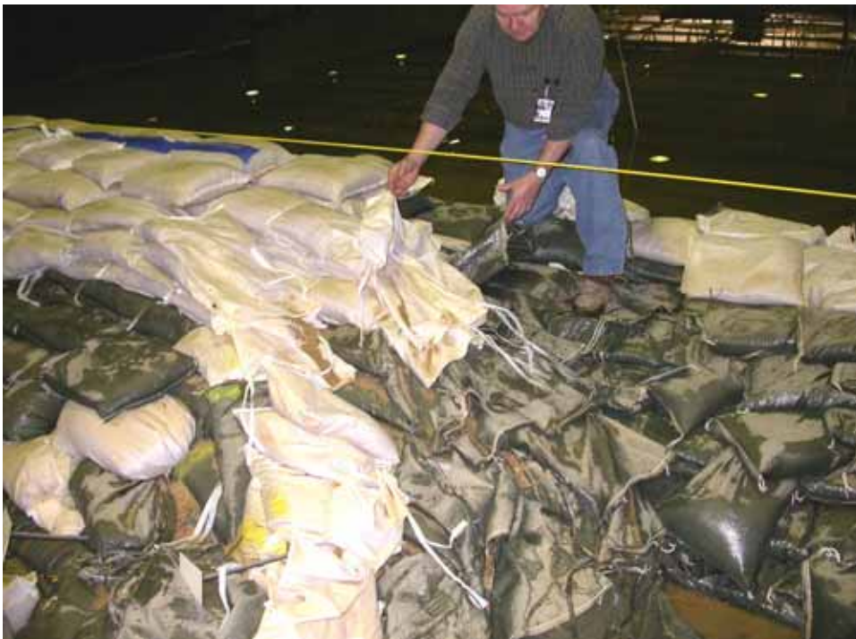
Figure 2-40. Sandbag levee autopsy after overtopping
