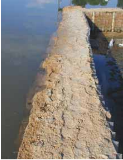
Figure 3-128. RDFW structure before overtopping
