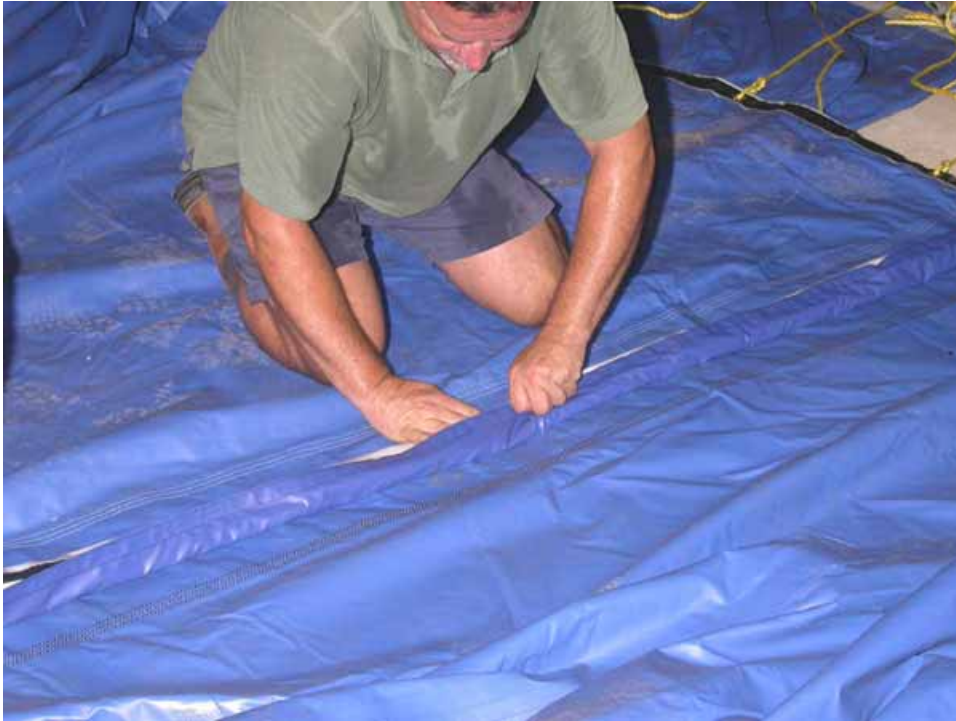
Figure 2-204. Vinyl tarp seam connection complete
