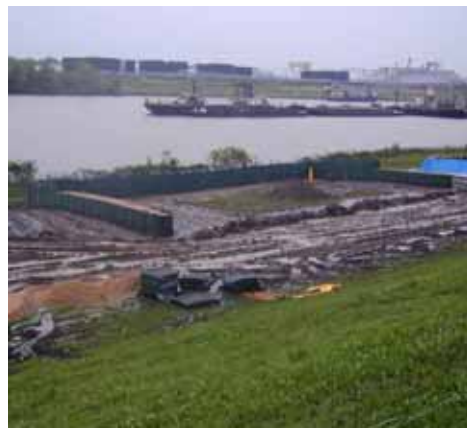
Figure 3-79. Completed structure from protected side
