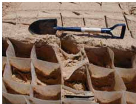
Figure 3-136. Shovel used to remove sand
