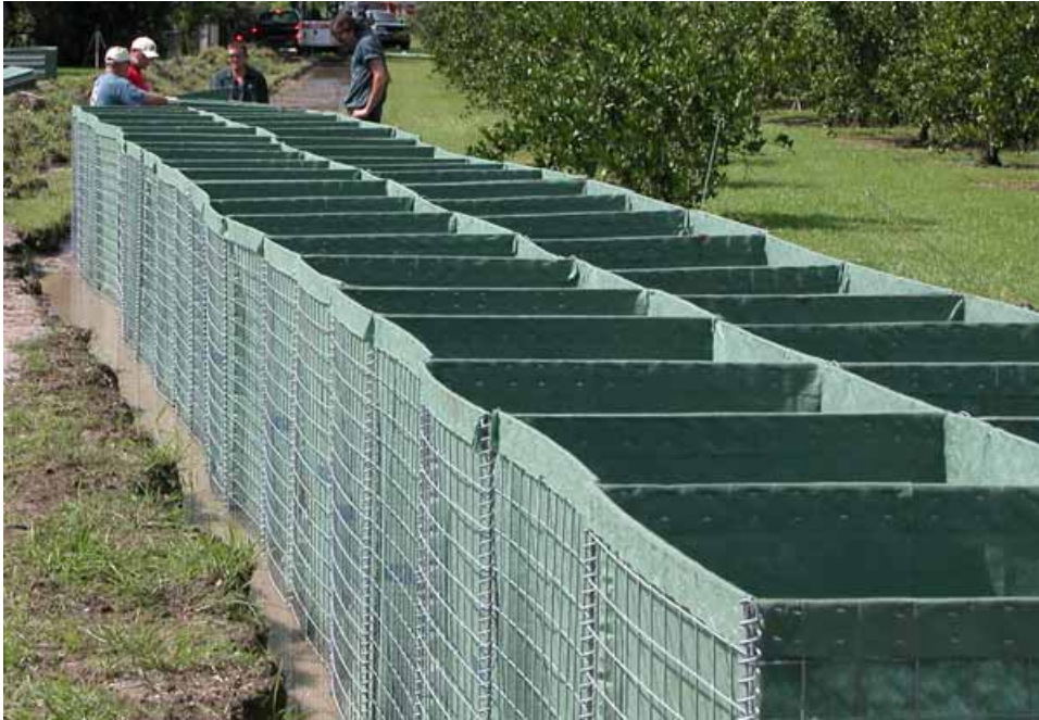
Figure 2-44. Hesco Bastion Concertainer® basket units, assembled and empty
