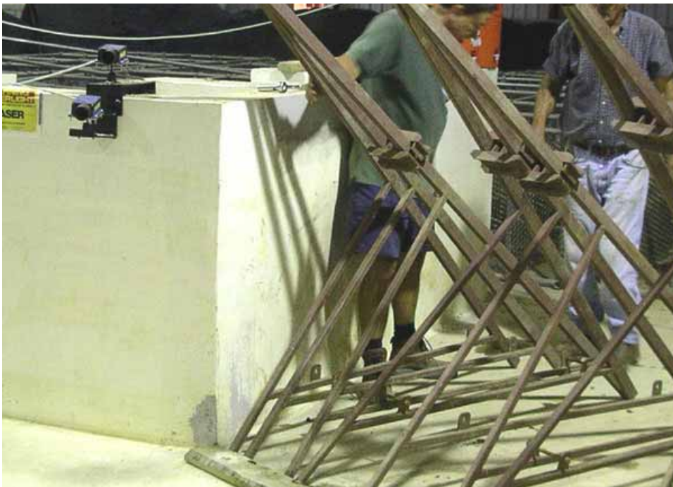
Figure 2-192. Frame installation against heel stop from left abutment wall
