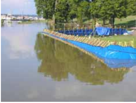
Figure 3-164. 10 June 2004, 3.5 ft of water against structure
