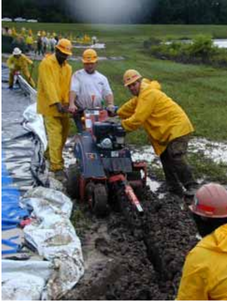
Figure 3-152. Excavating trench for liner leading edge
