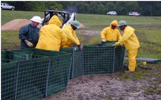
Figure 3-70. Installation of base row units
