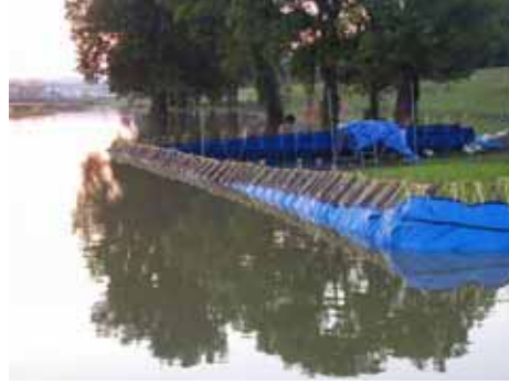
Figure 3-165. 11 June 2004, structure overtopped
