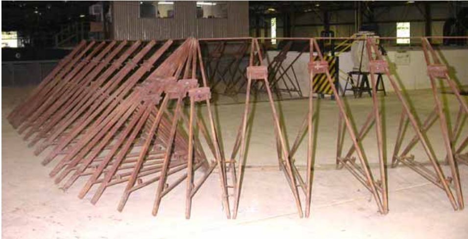
Figure 2-196. Completed frame assembly
