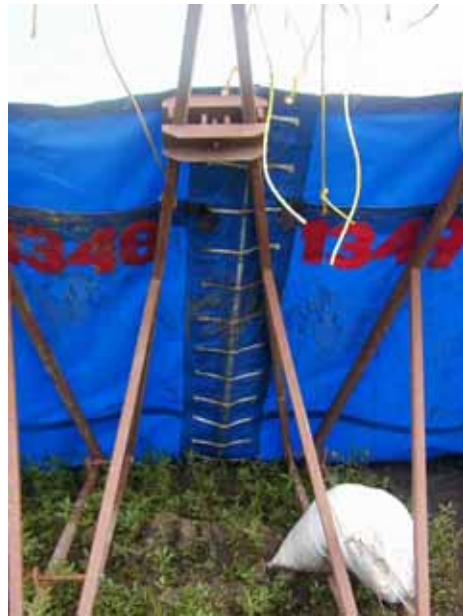
Figure 3-150. Seam between liner membrane sections
