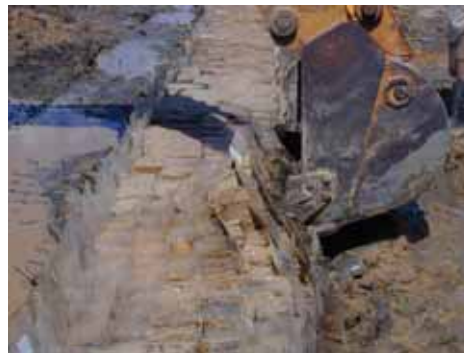
Figure 3-142. Removal with backhoe
