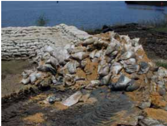
Figure 3-61. Removal of east tieback section
