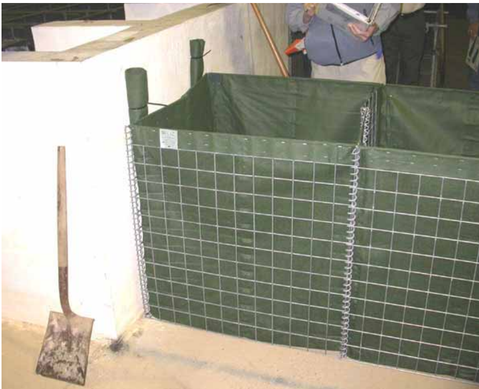
Figure 2-51. Right concrete wall abutment
