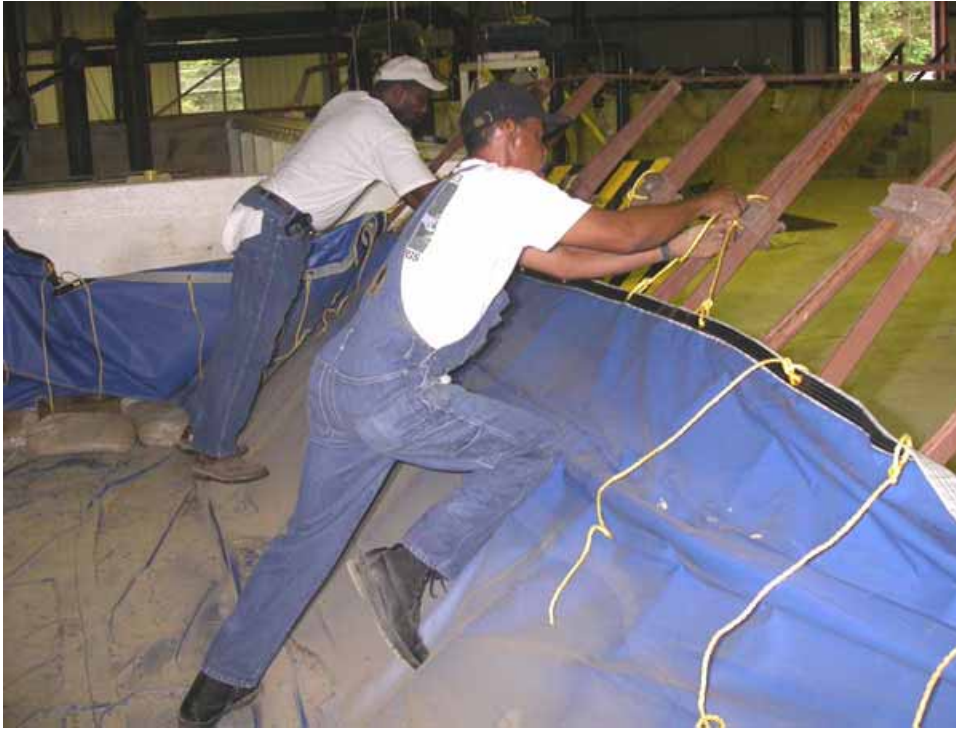
Figure 2-246. Removing vinyl tarp ties from frame
