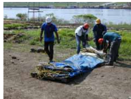
Figure 3-187. Rolling folded liner
