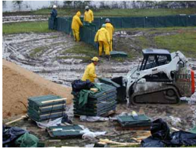
Figure 3-73. Construction of base row tieback section
