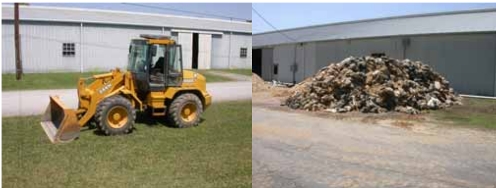
Figure 2-43. Heavy equipment used to disassemble sandbags and waste sandbags
