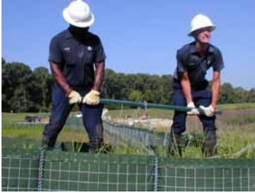
Figure 3-93. Removing center connection pins
