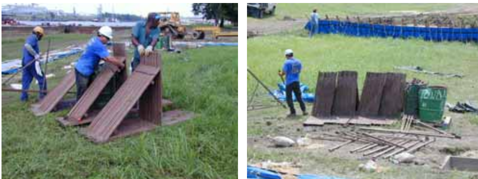
Figure 3-182. Removal staging area
