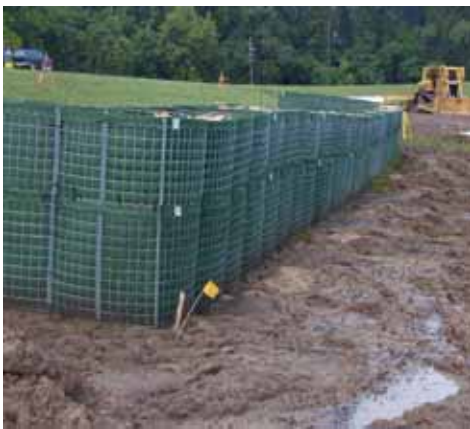
Figure 3-78. Riverward face of completed structure
