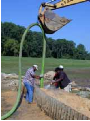
Figure 3-139. Vacuuming sand
