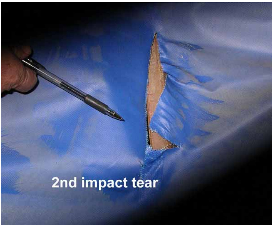
Figure 2-242. View of gash caused by large log. Note frame member behind slit
