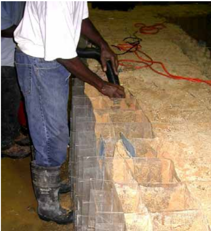
Figure 2-168. Removing sand using vacuum cleaner
