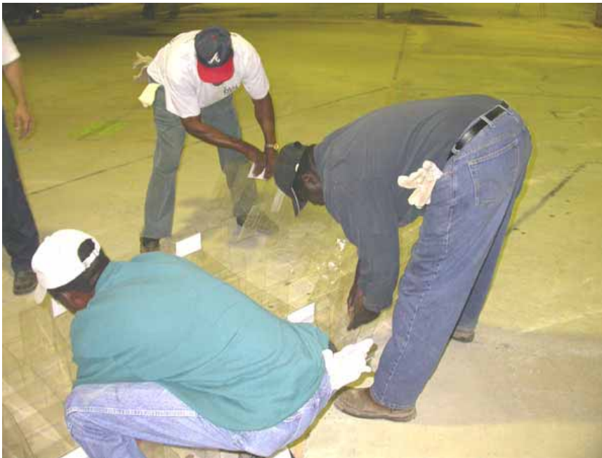
Figure 2-102. Laying expanded grid unit on floor
