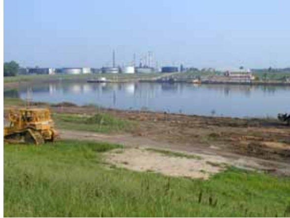
Figure 3-66. Structure completely removed
