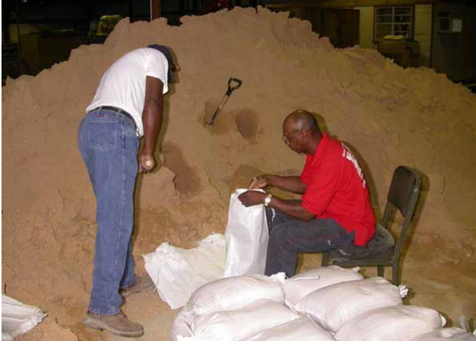
Figure 2-187. Apron sandbag filling operation
