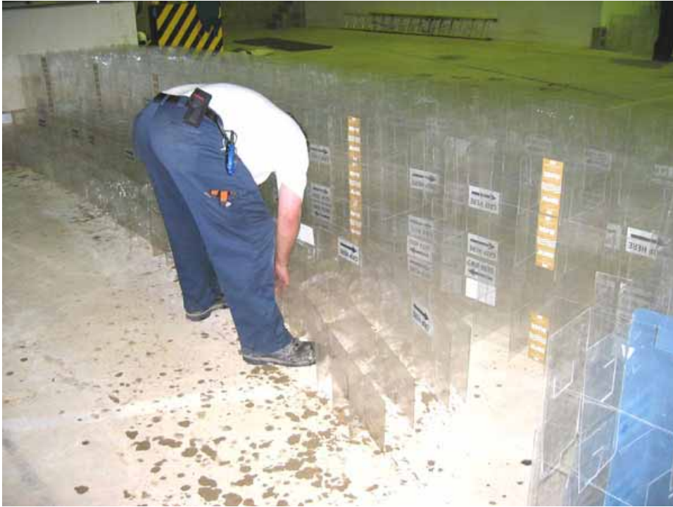
Figure 2-111. Installation of toe grid on pool side of right wall
