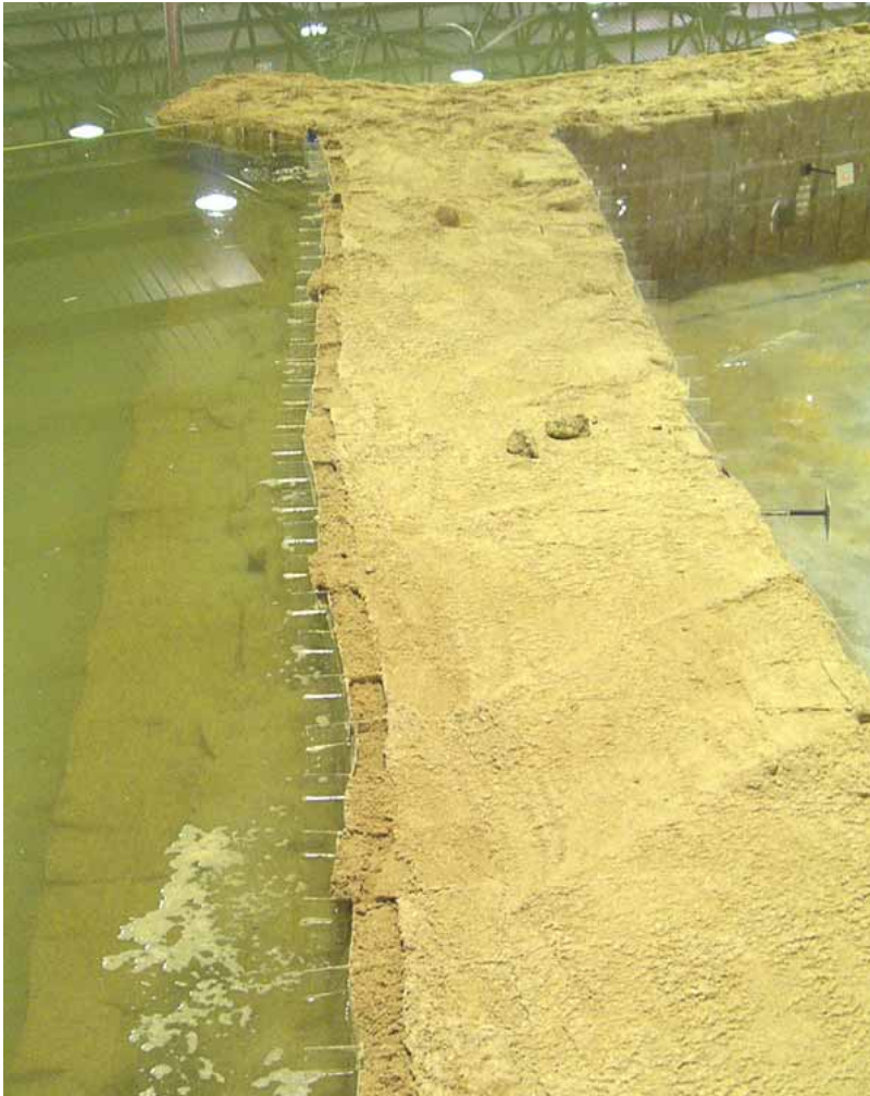
Figure 2-136. View looking down left wall
