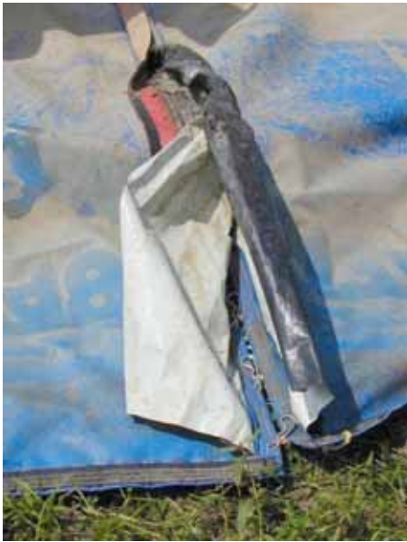
Figure 3-183. Disconnecting two sections of liner
