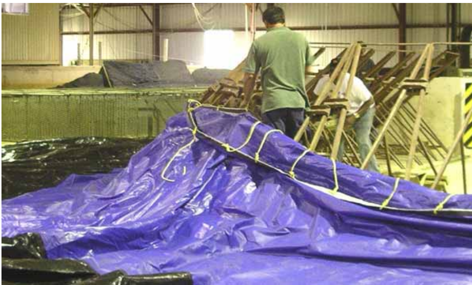
Figure 2-205. Pulling vinyl tarp up to frame
