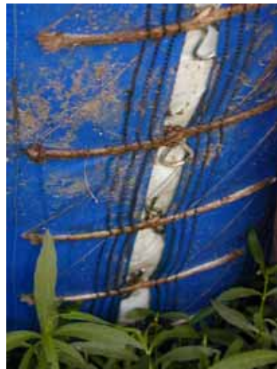
Figure 3-173. Stressed liner seam
