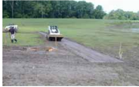
Figure 3-106. RDFW site back-dragged prior to construction
