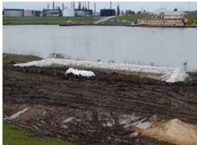
b. From protected side
