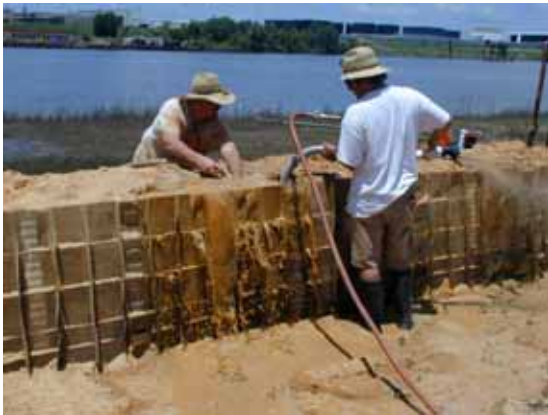
Figure 3-133. Hand-held vacuum device and water hose (saturated sand)
