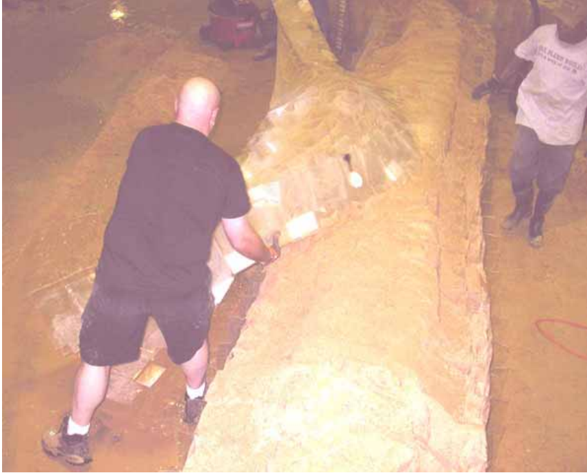
Figure 2-175. Removing grid units from wall
