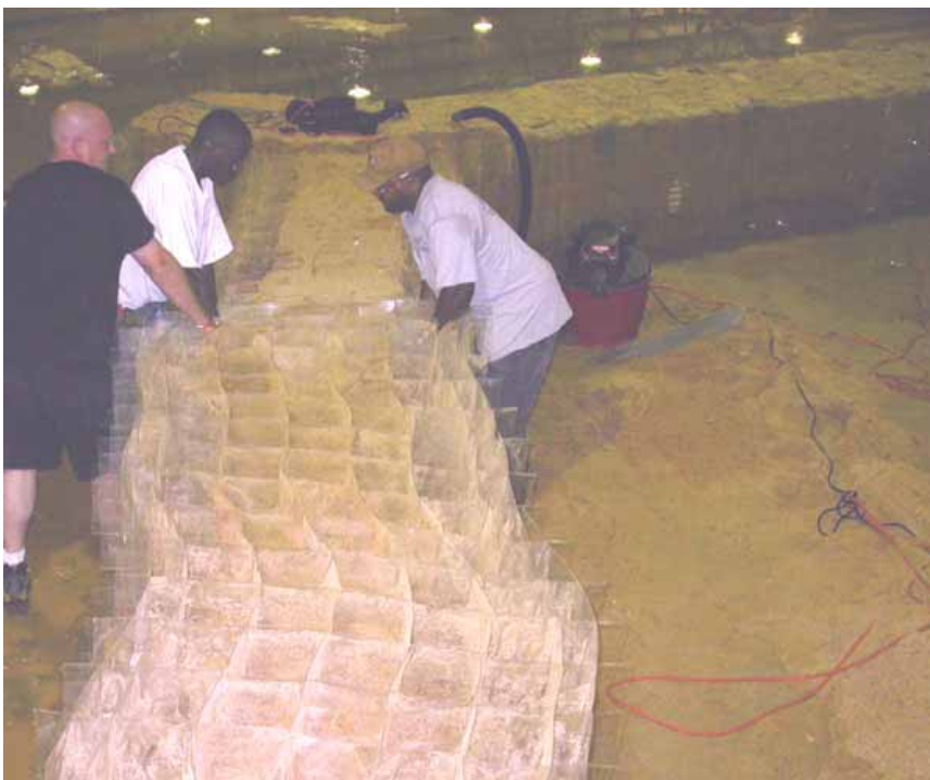
Figure 2-174. Loosening attached grid units
