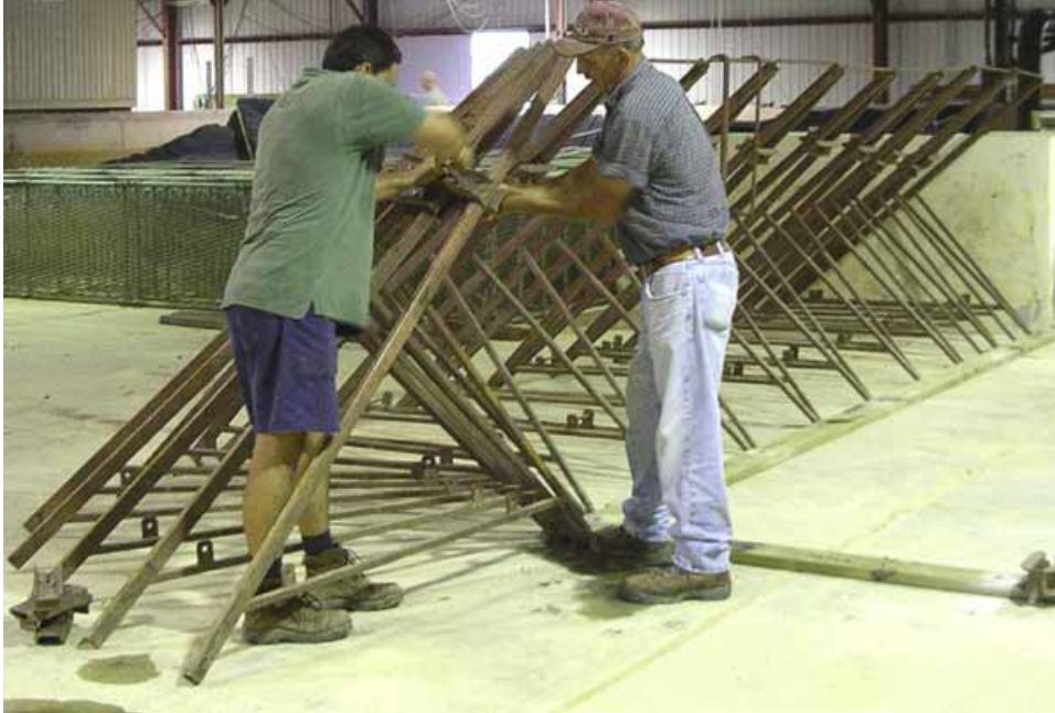
Figure 2-194. Installing frame at 90-deg corner
