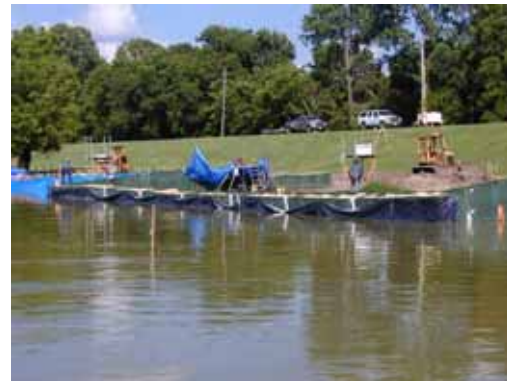
Figure 3-85. 9 June 2004, 3.1 ft of water against structure
