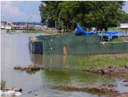
Figure 3-84. 8 June 2004, 2.7 ft of water against structure
