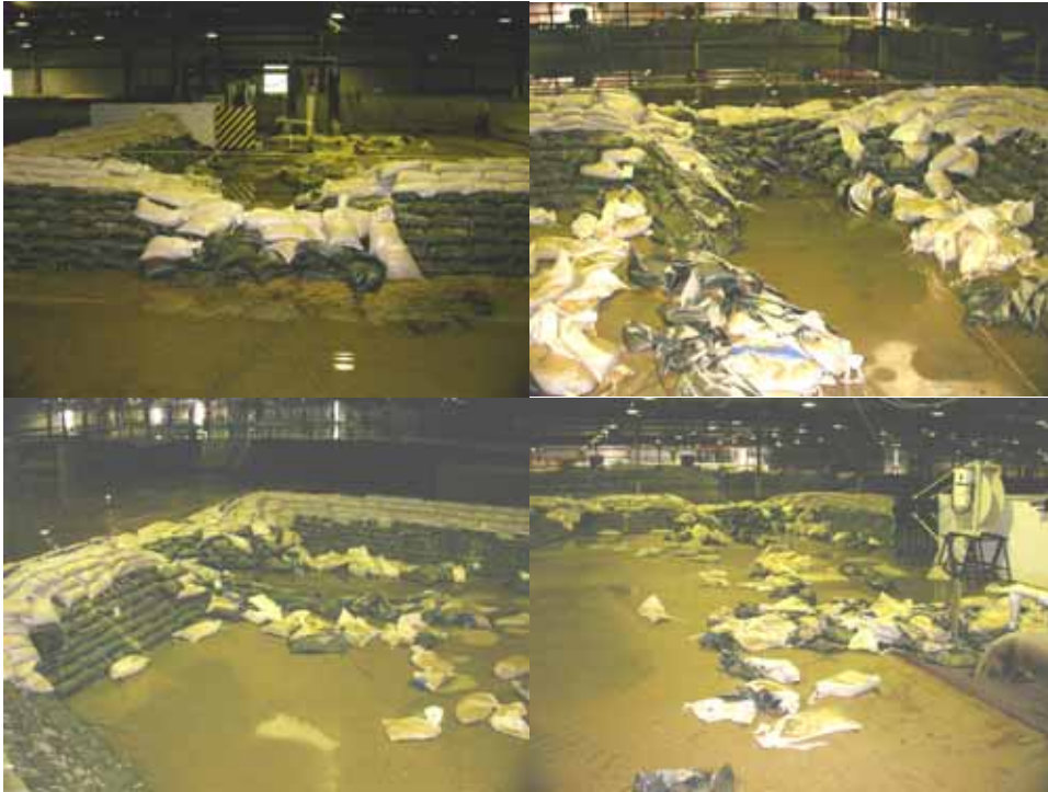
Figure 2-39. Sandbag levee after failure
