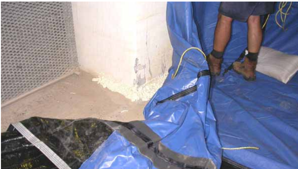
Figure 2-209. Expandable foam treatment at concrete wall abutment
