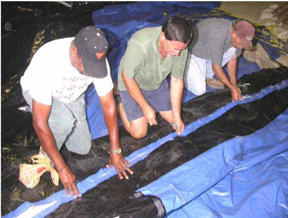
Figure 2-201. Securing two tarp sections together with hairpin cotters
