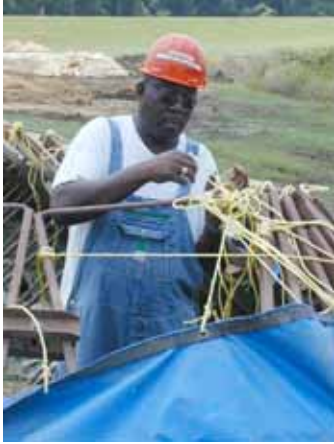
Figure 3-178. Removing liner membrane from supporting frame
