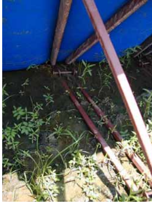
b. Sunken frame along riverward face
