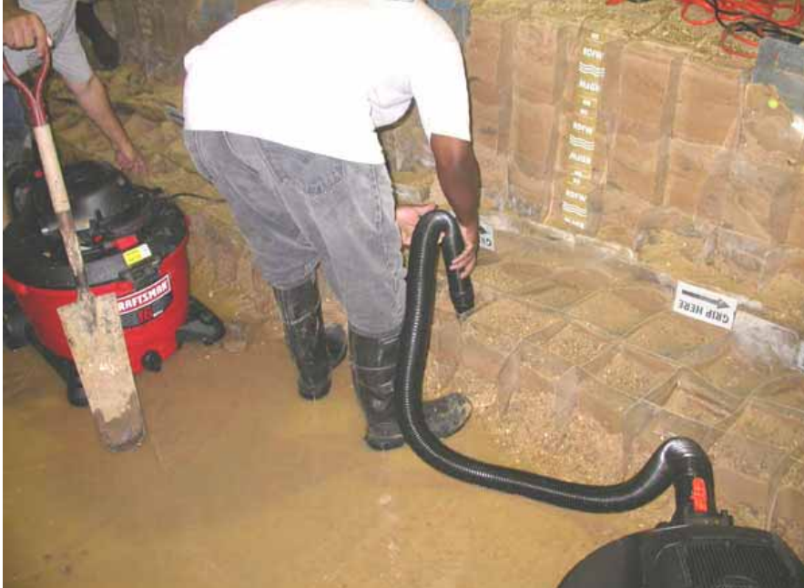
Figure 2-163. Vacuuming sand out of toe grid units
