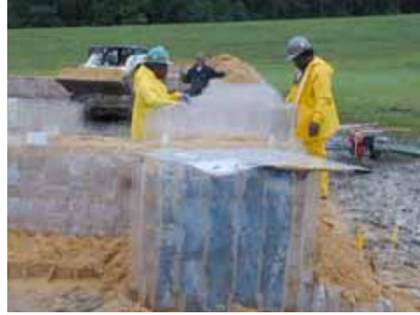
Figure 3-114. Installation of top row units (required raise)
