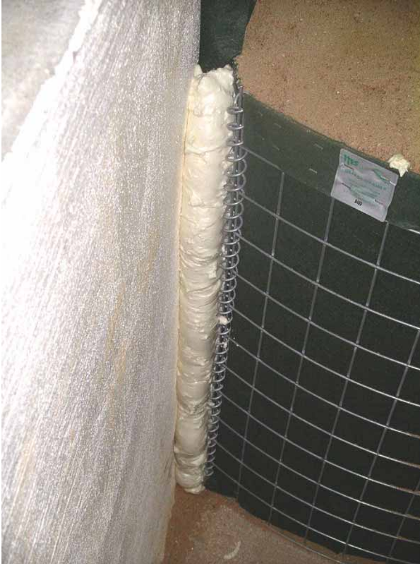
Figure 2-59. Expanded foam at abutment with concrete wall
