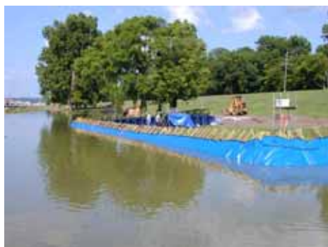
Figure 3-163. 9 June 2004, 3.1 ft of water against structure
