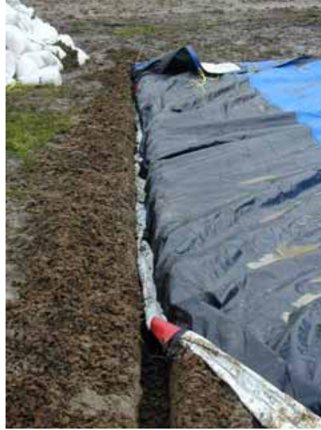
Figure 3-153. Liner leading edge placed in trench
