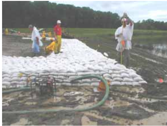
Figure 3-41. Measuring the height of structure
