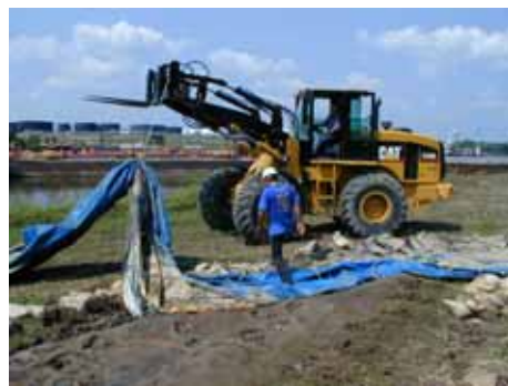
Figure 3-185. Forklift removing liner from excavated trench
