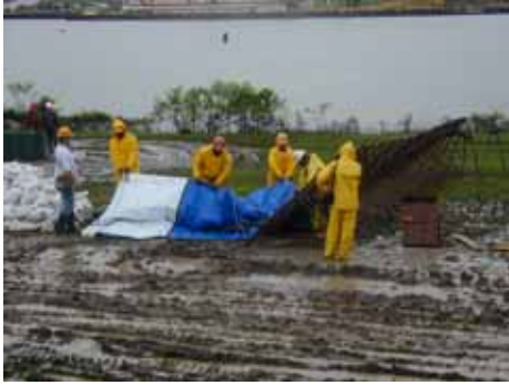
Figure 3-149. Unrolling liner membrane
