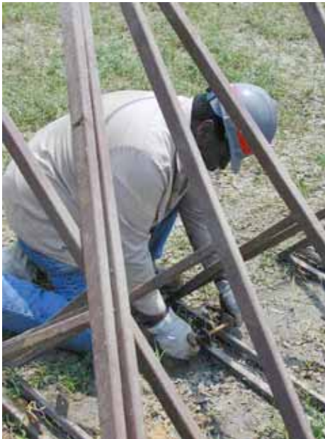
Figure 3-179. Disassembling supporting frame (bolts and clamps)
