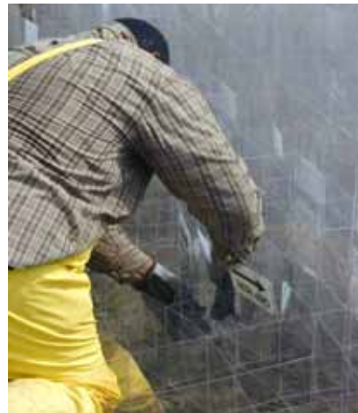
Figure 3-108c. Interlocking of RDFW units
