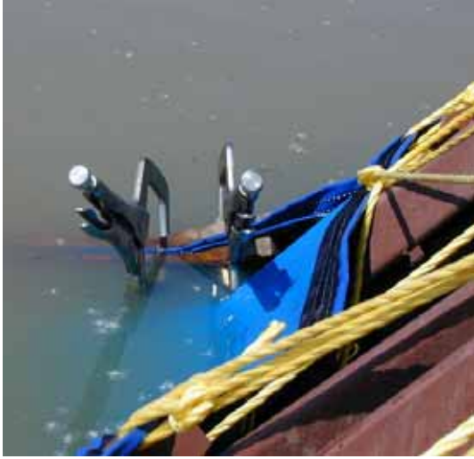
Figure 3-169. Sagging liner repair (repair 2)
