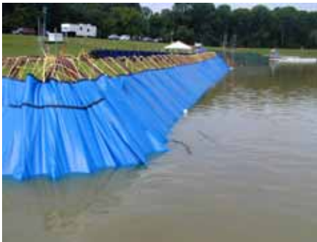
Figure 3-160. 6 June 2004, 1.3 ft of water against structure
