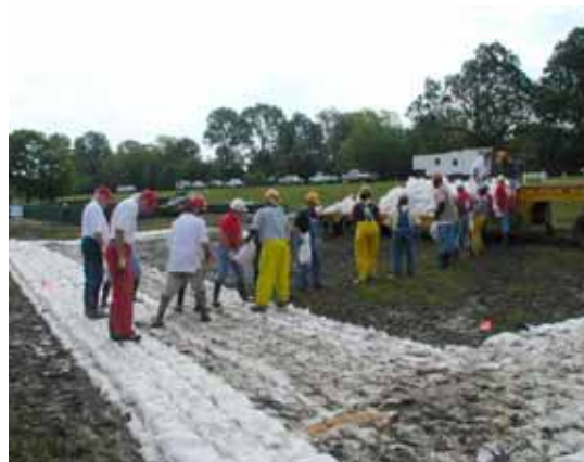
b. Laborers passing sandbags
