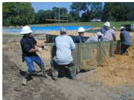
Figure 3-99. Removal of base row half units
