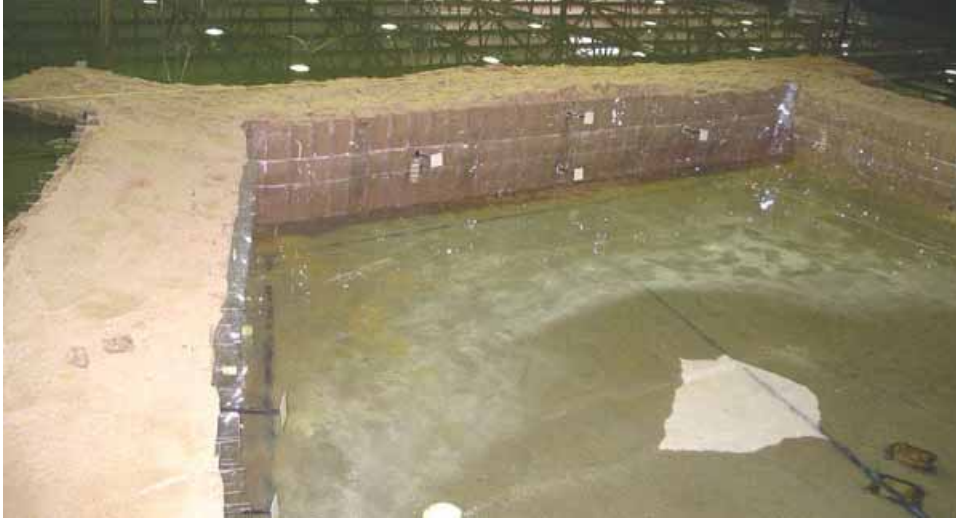
Figure 2-135. View of seepage under structure
