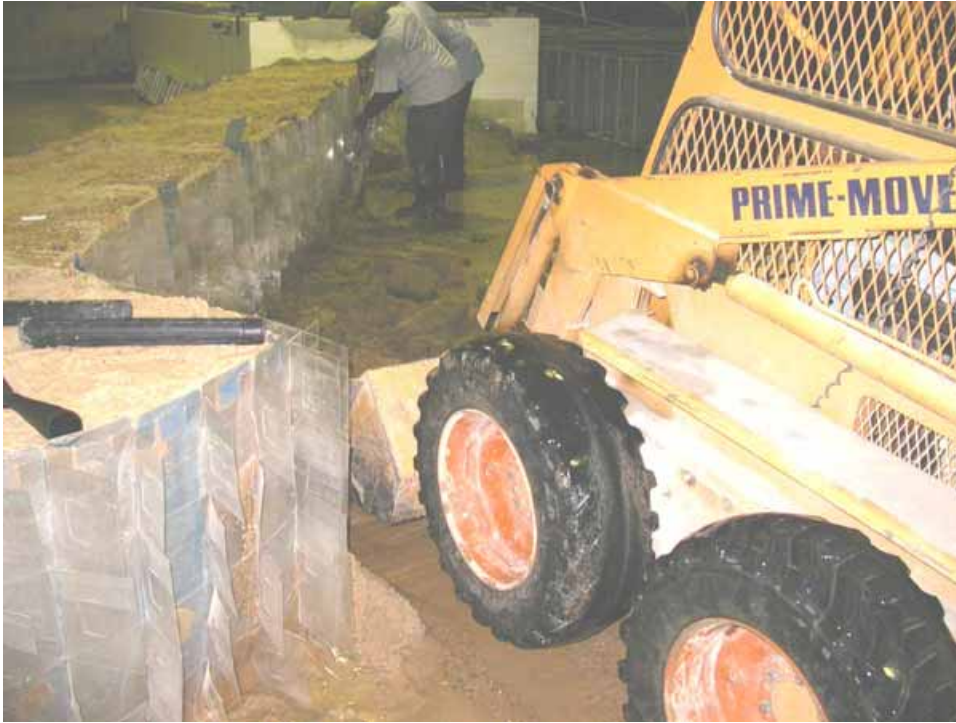
Figure 2-165. Removing toe grid materials
