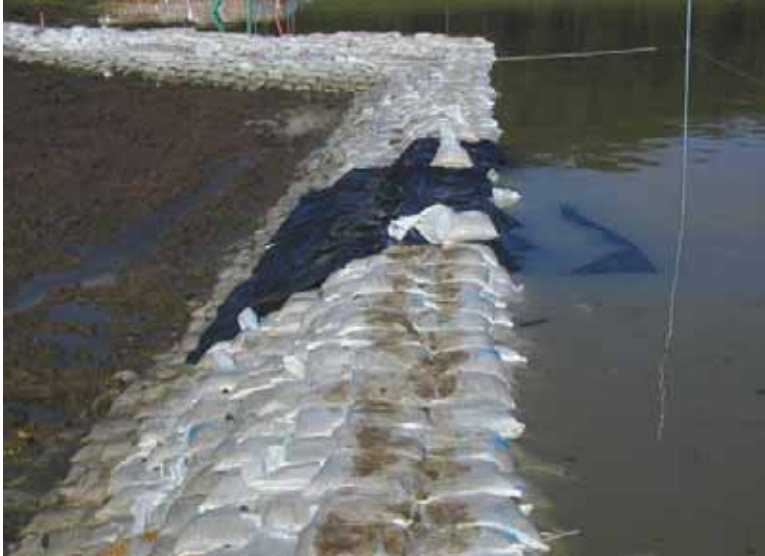
Figure 3-56. Plastic sheeting over riverward face
