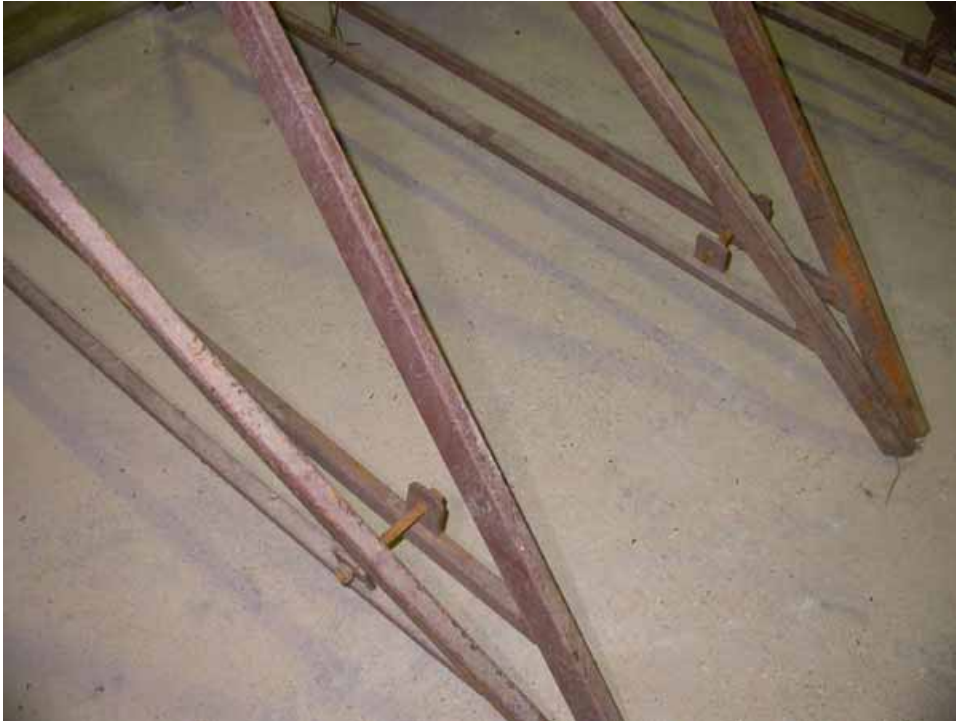
Figure 2-189. Connection at lower leg of frames
