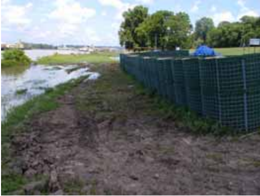
Figure 3-80. 4 June 2004, no water against structure
