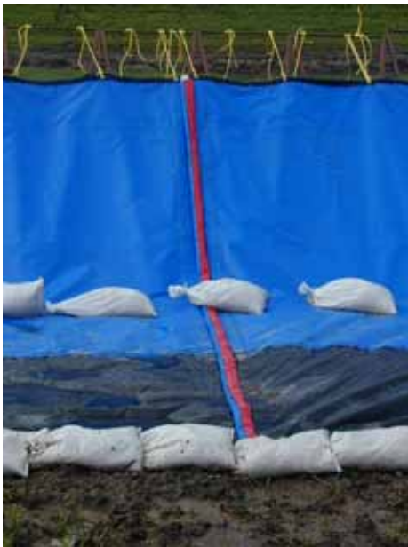
Figure 3-150. Seam between liner membrane sections
