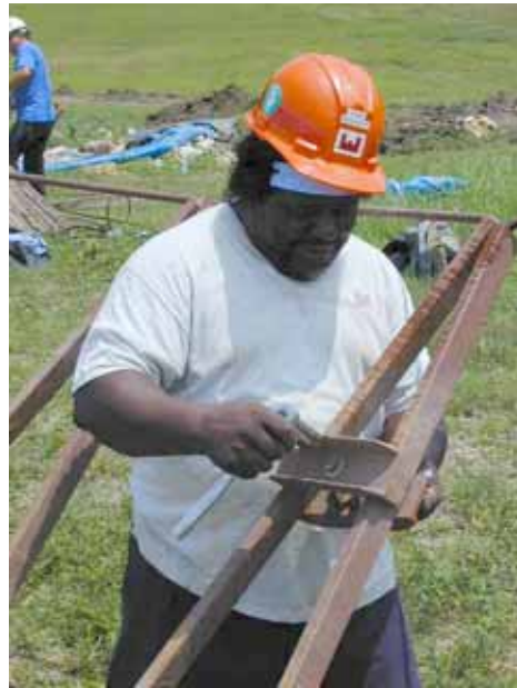
Figure 3-179. Disassembling supporting frame (bolts and clamps)
