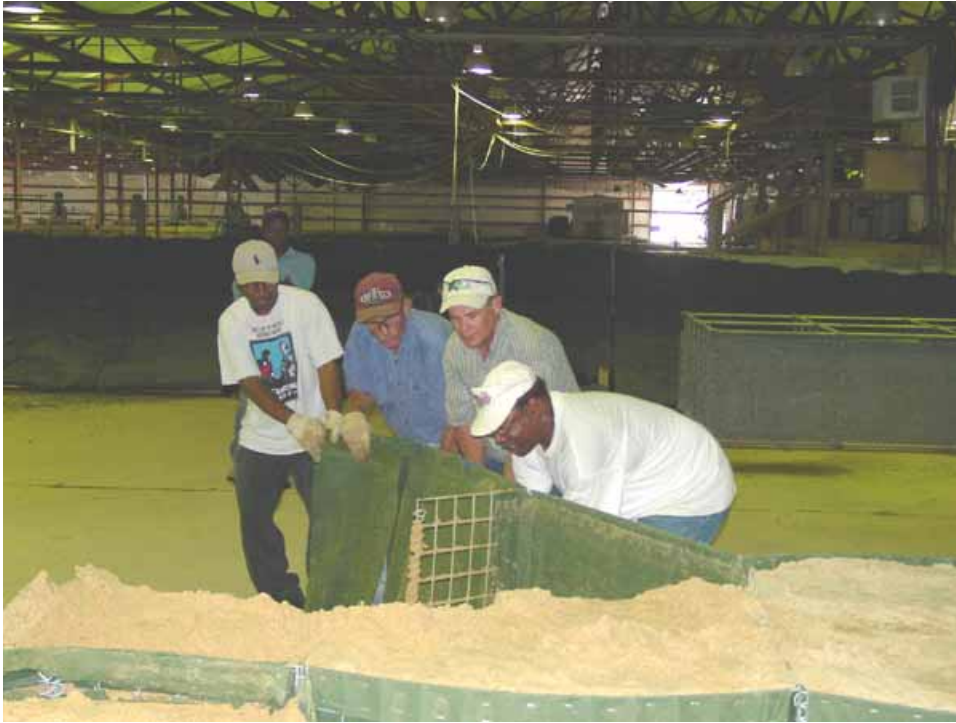
Figure 2-93. Pulling unit apart
