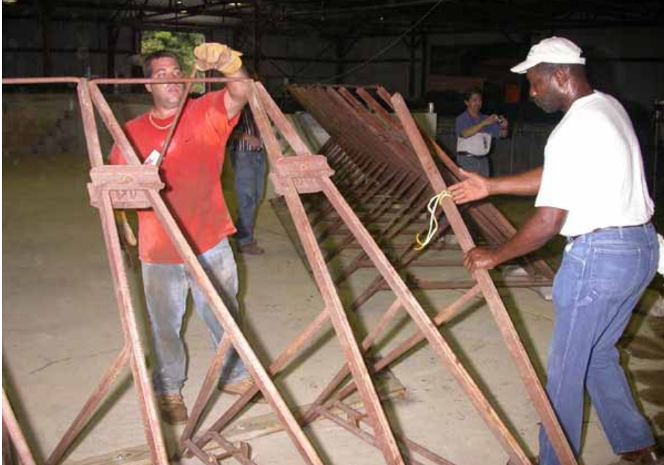
Figure 2-250. Removing top bars for frame removal
