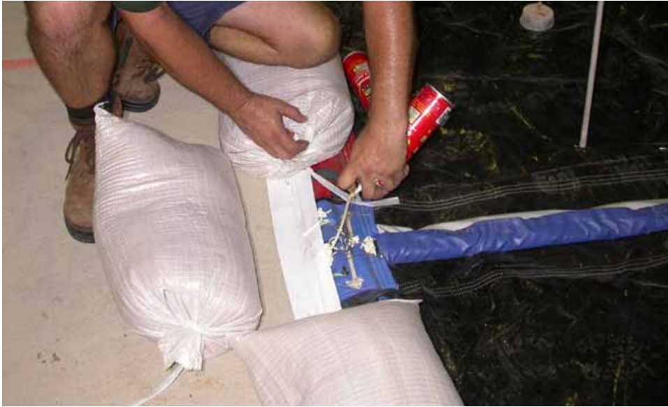
Figure 2-208. Expandable foam treatment at vinyl tarp apron edge
