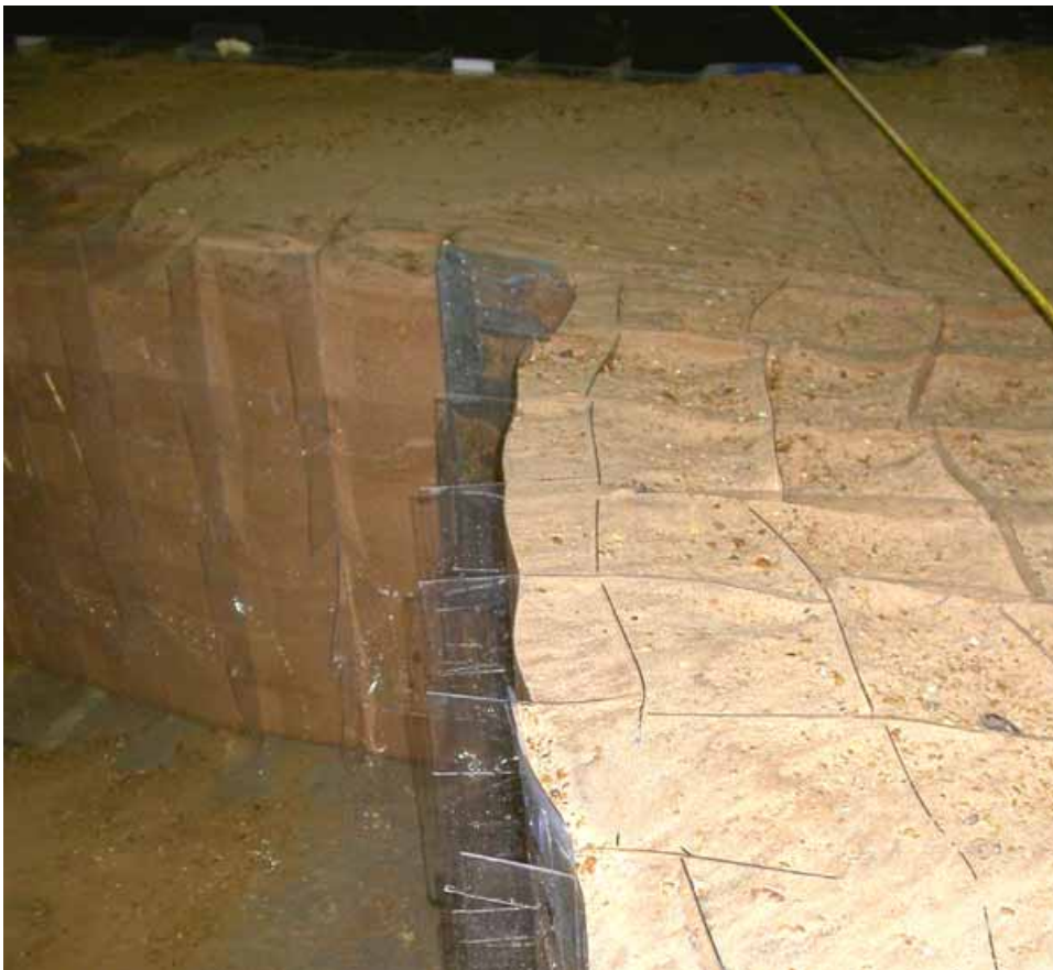
Figure 2-155. Close-up at intersection of left and center walls
