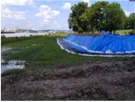
Figure 3-158. 4 June 2004, no water against structure
