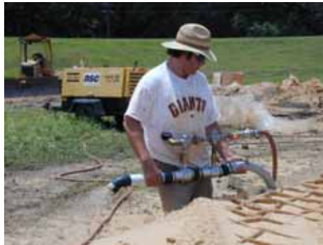
Figure 3-132. Hand-held vacuum device (consolidated sand)
