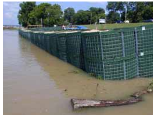
Figure 3-83. 7 June 2004, 2.1 ft of water against structure
