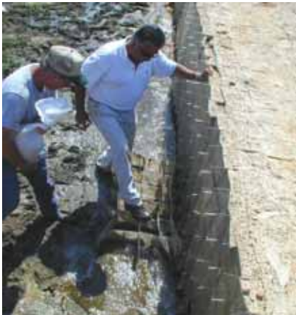
Figure 3-126. Using RDFW unit to contain sand boil
