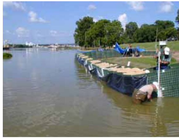
e. Packing bentonite into pipes
