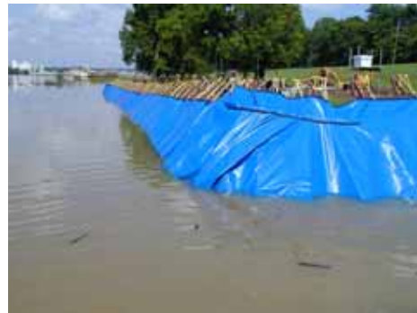
Figure 3-161. 7 June 2004, 2.1 ft of water against structure
