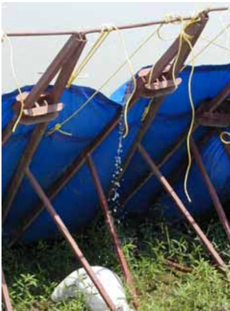
Figure 3-167. Sagging liner
