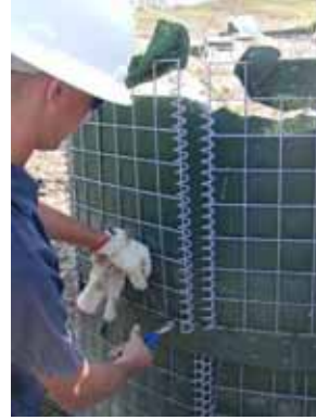
Figure 3-94. Removing zip ties
