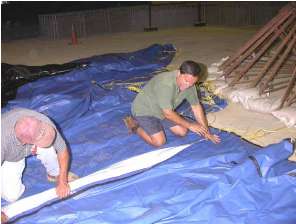
Figure 2-203. Hook and loop fastening seam flap
