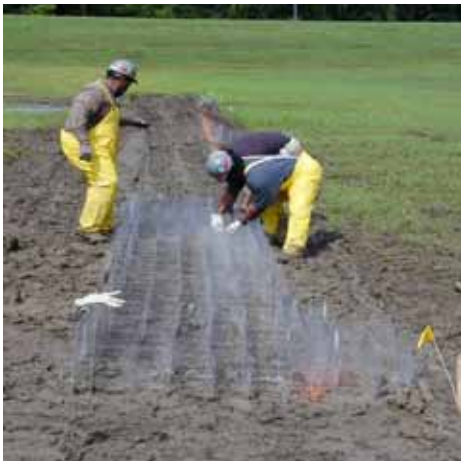
Figure 3-108b. Installation of RDFW base row
