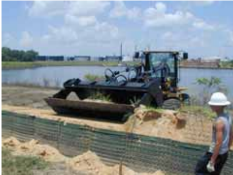
Figure 3-97. Removal of top row sand
