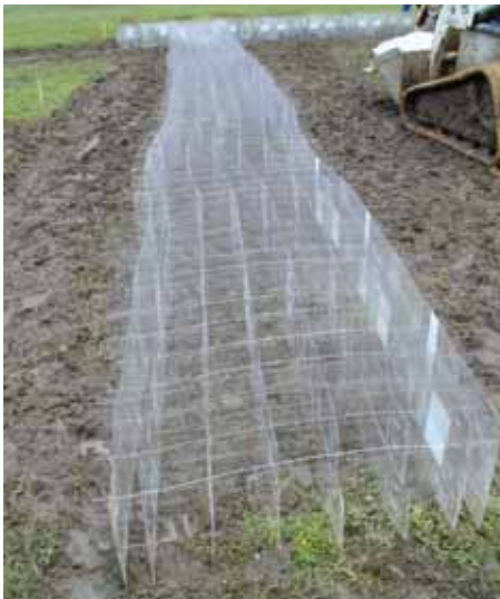
Figure 3-111. Stair-stepped tieback section
