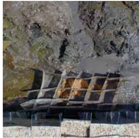
Figure 3-127. Contained sand boil
