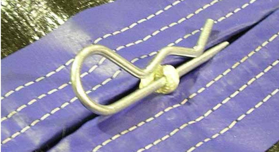
Figure 2-200. Hairpin cotter for securing two vinyl tarp sections together
