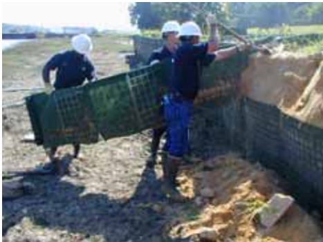
Figure 3-95. Removal of top row half units
