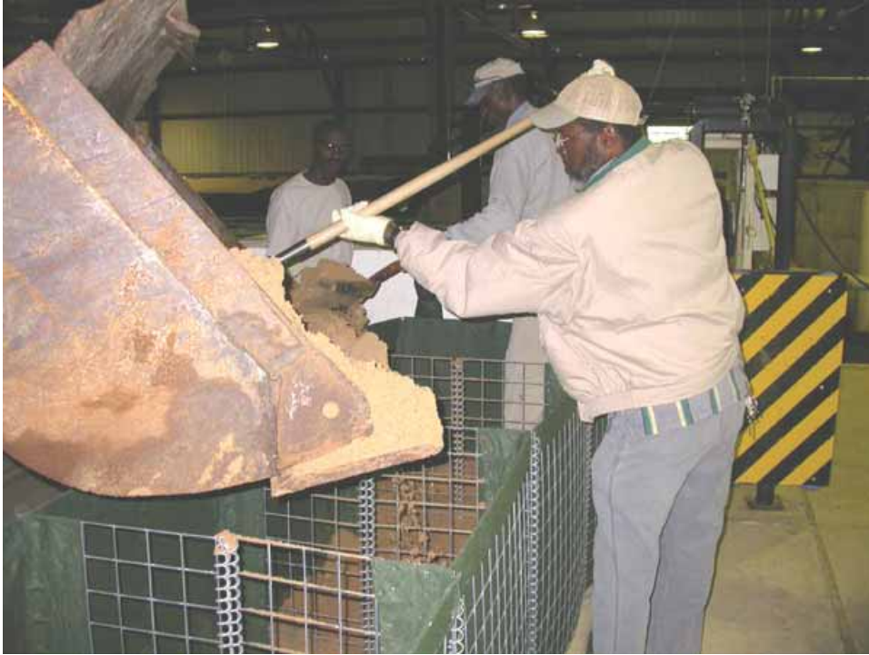
Figure 2-54. Shoveling sand into unit
