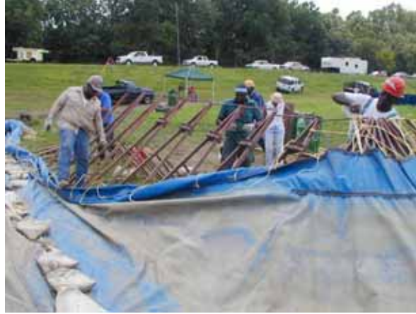
Figure 3-178. Removing liner membrane from supporting frame
