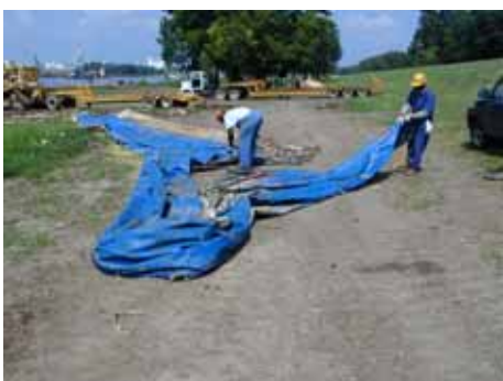
Figure 3-186. Folding liner
