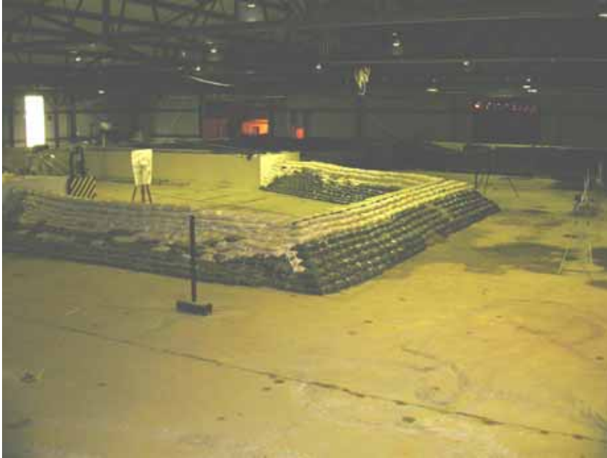
Figure 2-28. Sandbag levee after repair
