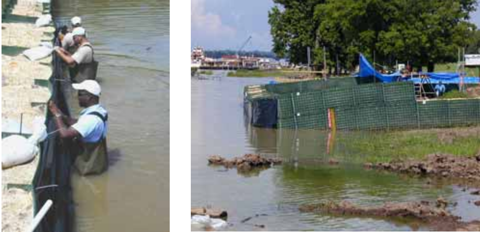
Figure 3-91. Attaching plastic sheeting to riverward face of Hesco Bastion structure
