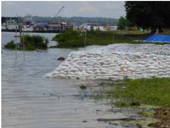
Figure 3-45. 4 June 2004, 1.0 ft of water against structure
