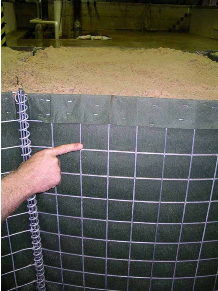
Figure 2-86. Log impact zone on center wall, pool side
