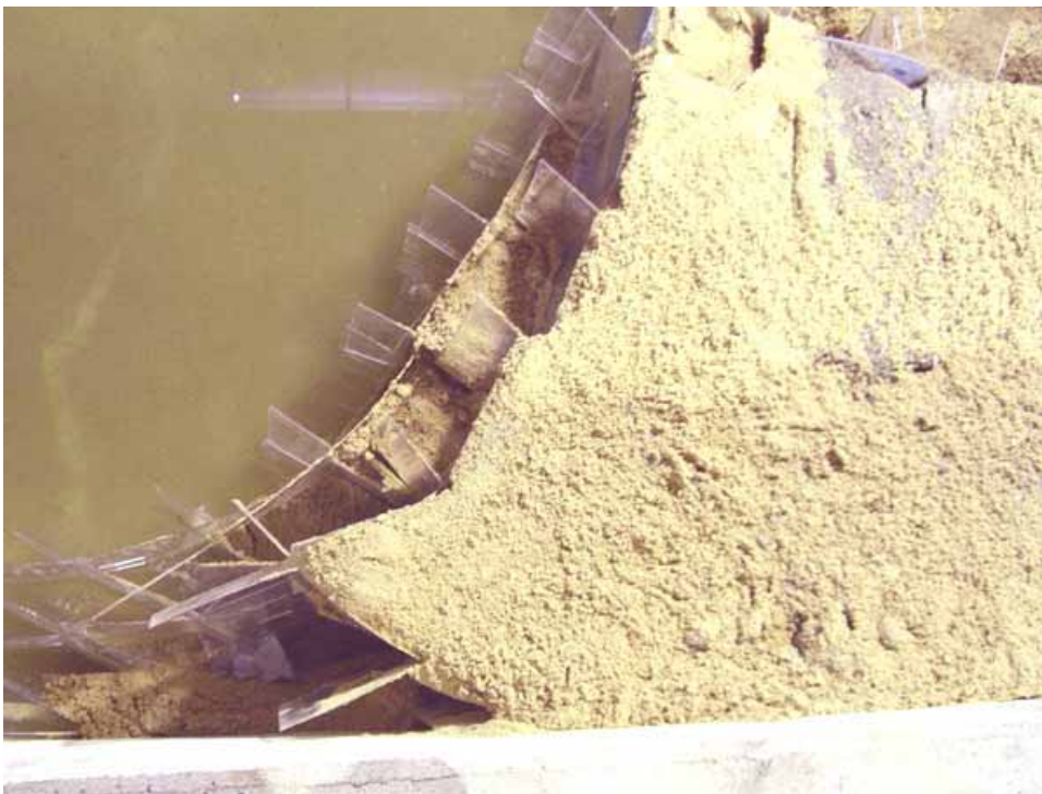
Figure 2-132. Left concrete wall abutment
