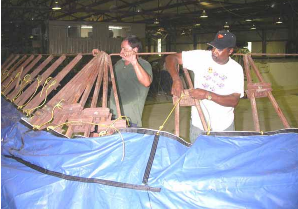
Figure 2-206. Tying tarp to frame
