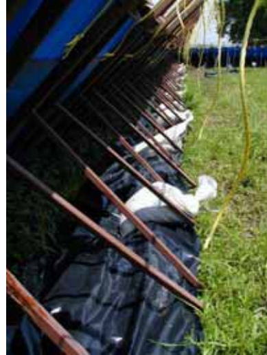
Figure 3-170. Typical preparation for overtopping (plastic sheeting)
