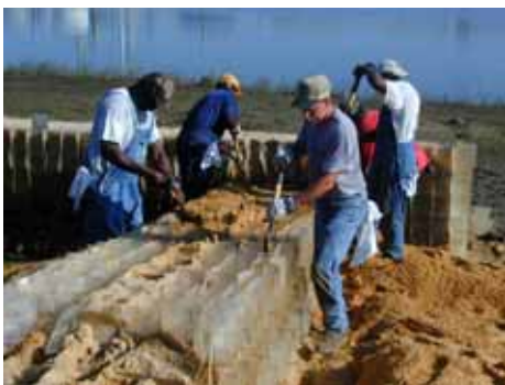
Figure 3-137. Removing sand with shovels
