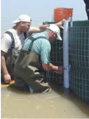
a. Attaching pipe to joints
