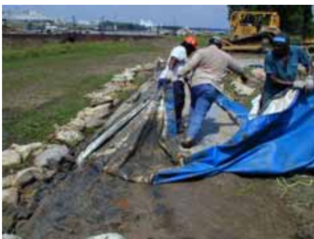
Figure 3-184. Laborers removing liner from excavated trench
