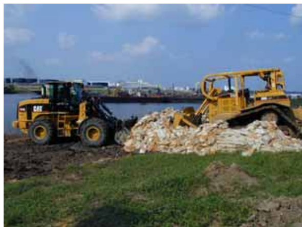
Figure 3-64. Dozer and front-end loader
