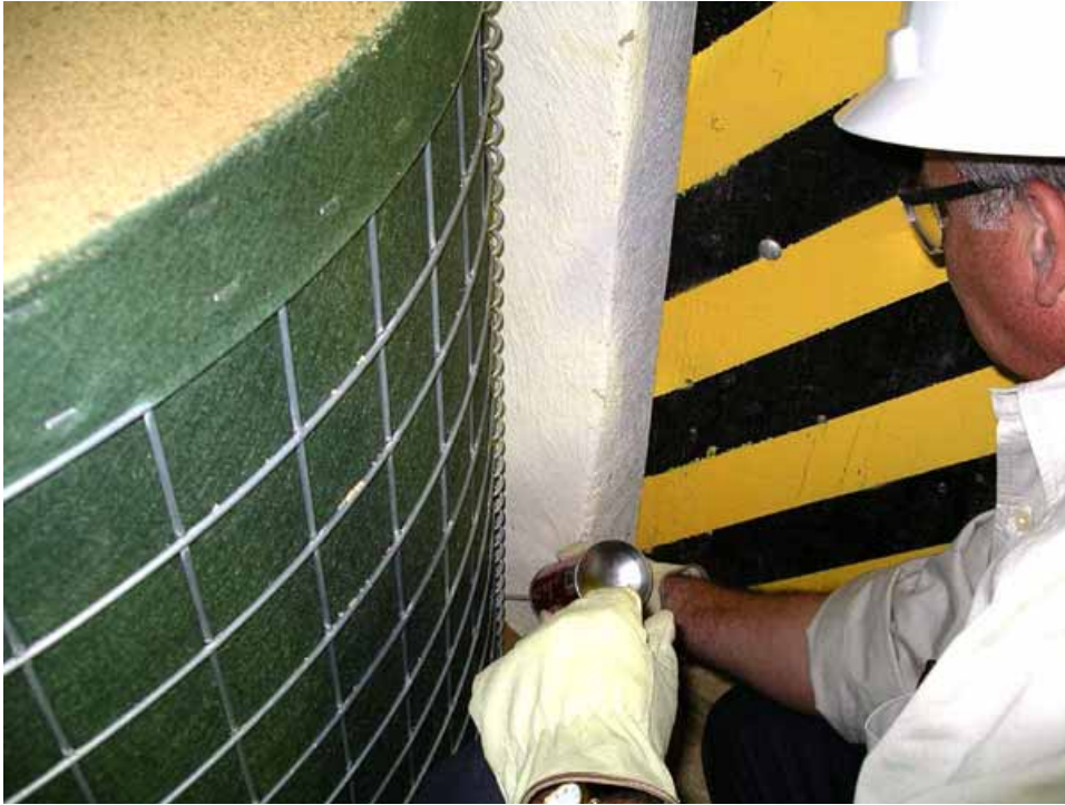
Figure 2-58. Sealing concrete wall abutment with aerosol foam
