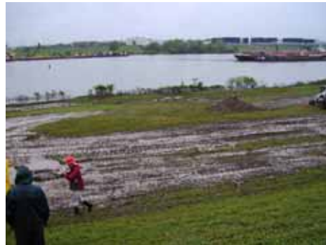
Figure 3-68. Hesco Bastion field site prior to construction
