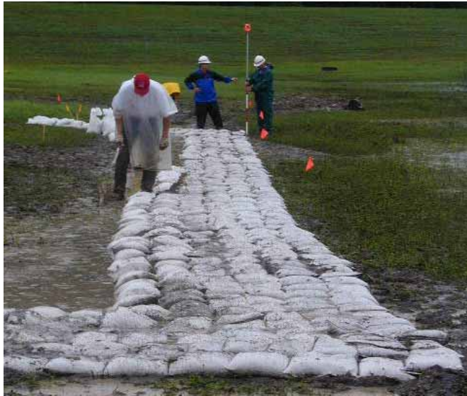
Figure 3-36. Partially completed riverward face, first row
