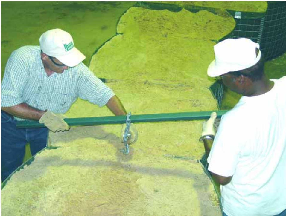
Figure 2-90. Preparing to remove center partition pin
