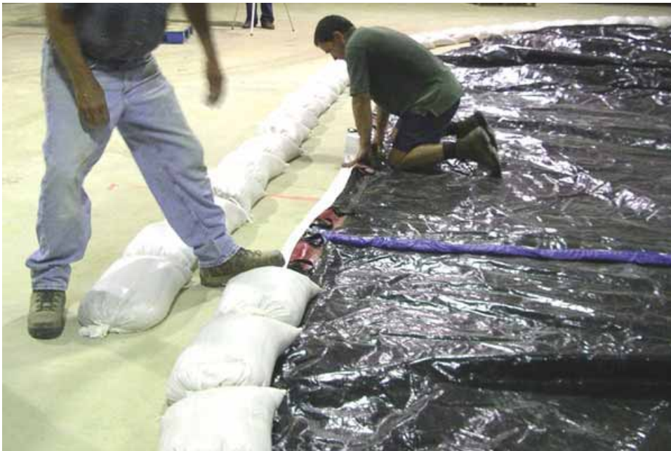
Figure 2-207. Taping apron to concrete floor and placing sandbags over tape
