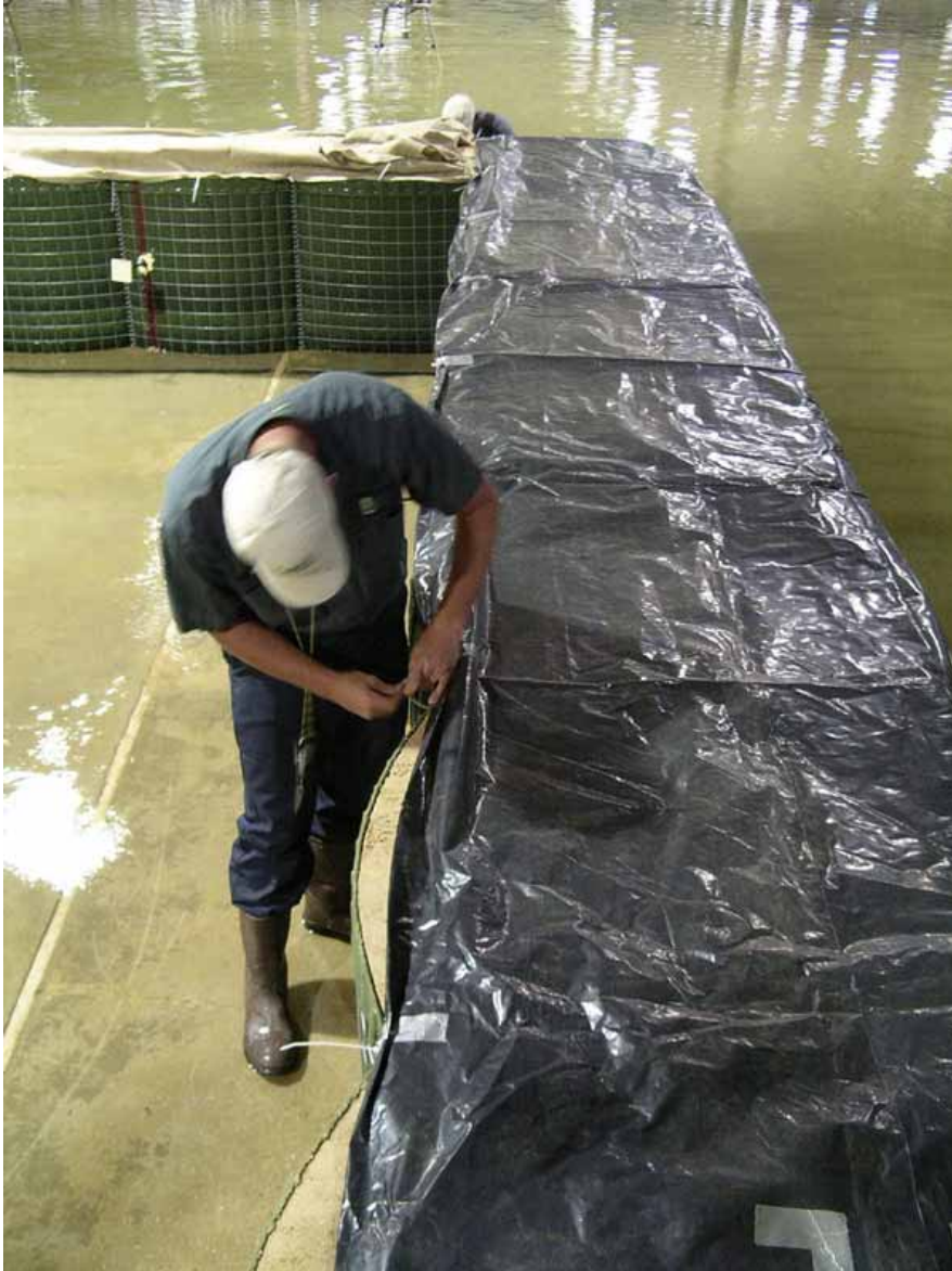
Figure 2-87. Repair 1, view along right wall
