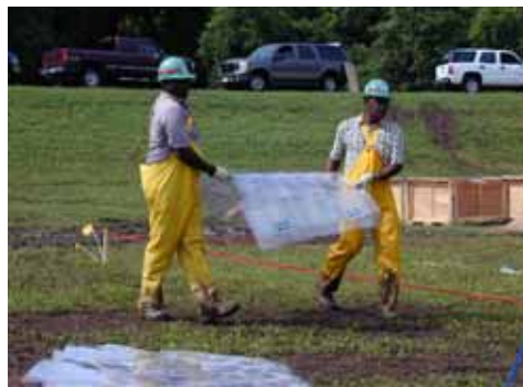
Figure 3-108a. Unpacking of RDFW units
