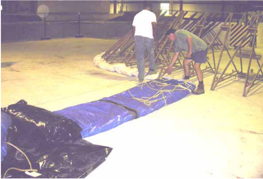
Figure 2-198. Unrolling tarp section
