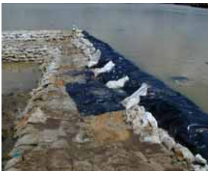
a. Prior to overtopping
