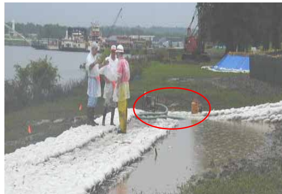
Figure 3-39. Water being pumped from structure
