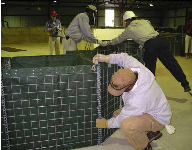
Figure 2-48. Pinning units together
