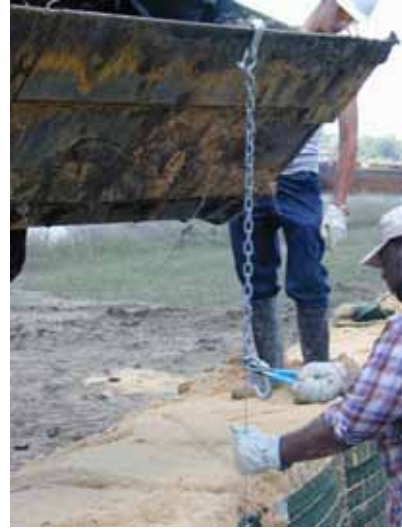
Figure 3-101. Removal of joint-connection pins with front-end loader
