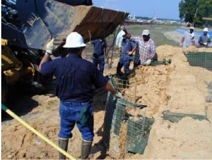
Figure 3-100. Removal of half units with front-end loader
