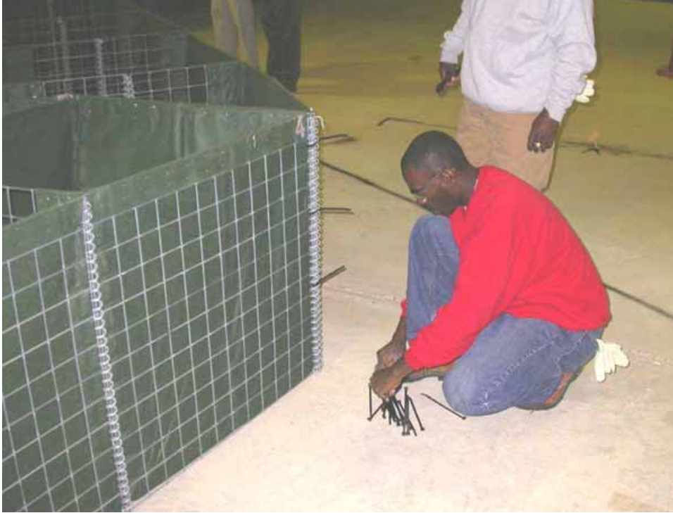
Figure 2-50. Cable ties at joint connections
