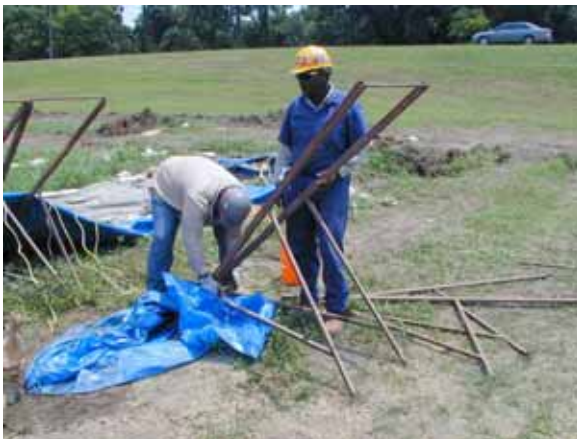
Figure 3-180. Disassembling supporting frame (members)
