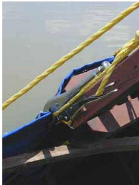
Figure 3-168. Sagging liner repair (repair 1)
