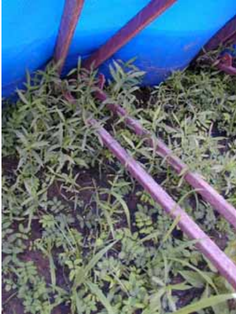
a. Unsunken frame along east tieback
