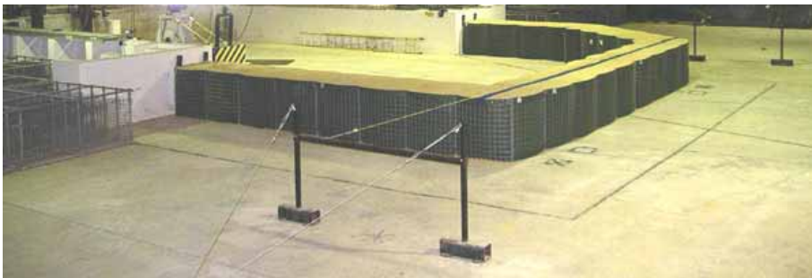
Figure 2-61. Center wall displacement monitoring system
