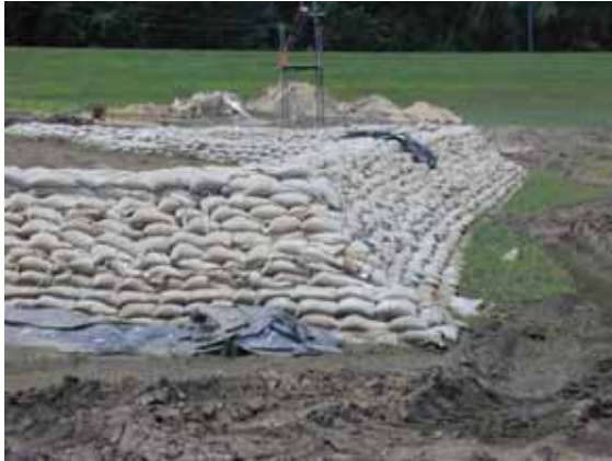
Figure 3-59. East side of structure
