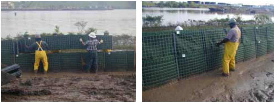
Figure 3-75. Installing top row units (required raise)
