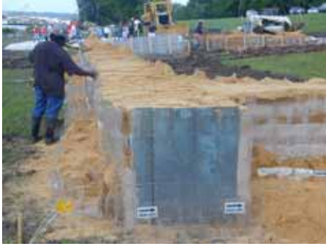
Figure 3-113. Filling of riverward face and east tieback section units
