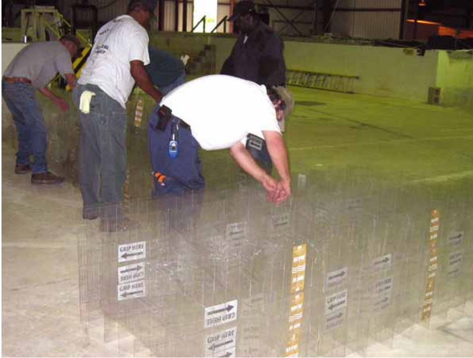
Figure 2-109. Third grid unit layer at right wall and center wall junction, viewed from pool side
